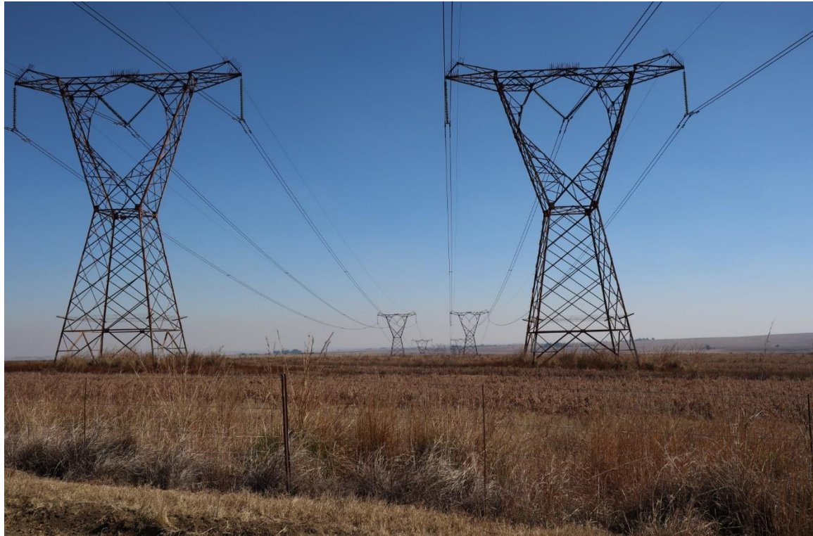
Plate 21, Camden / Sol 2 and the Camden / Tutuka 1 400kV power lines crossing the site are highly obvious as they cross ridgelines.
