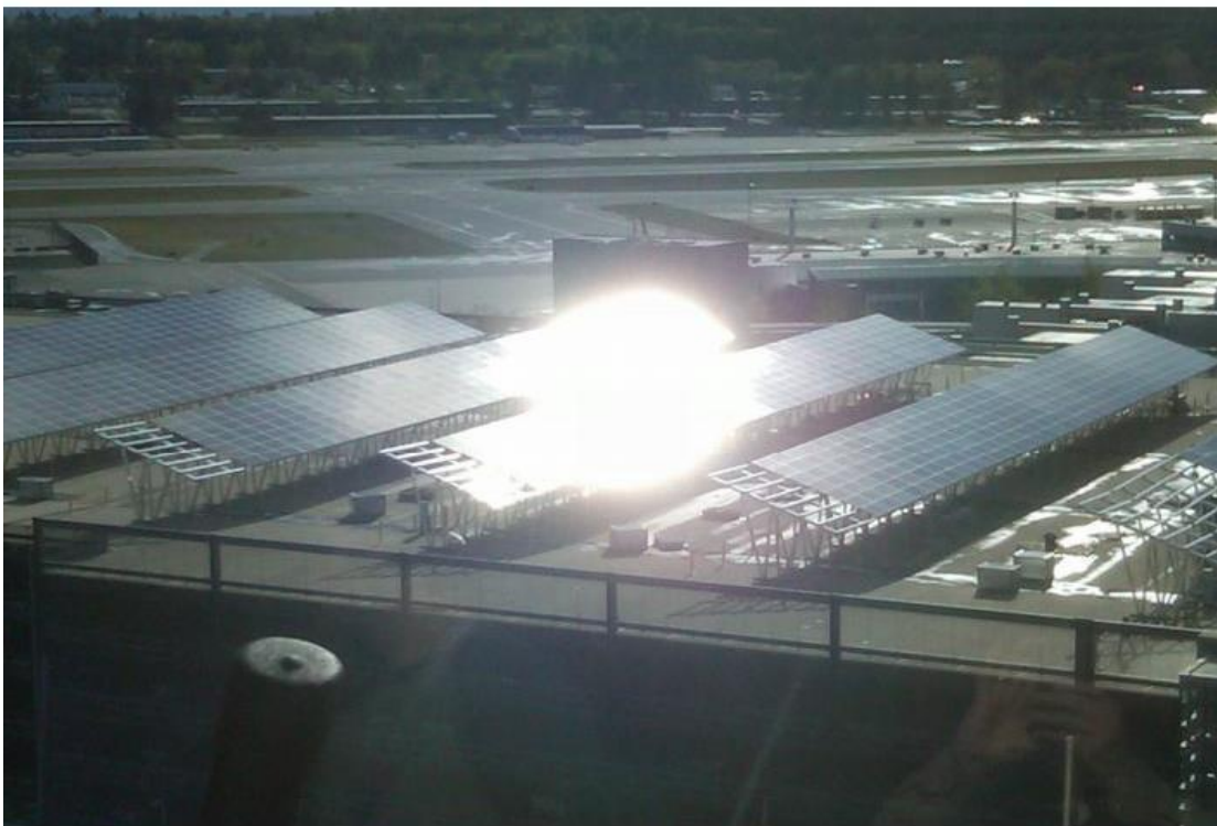
Plate 10 - Glare experienced in the Control Tower at Boston Regional Airport from an adjacent PV array
