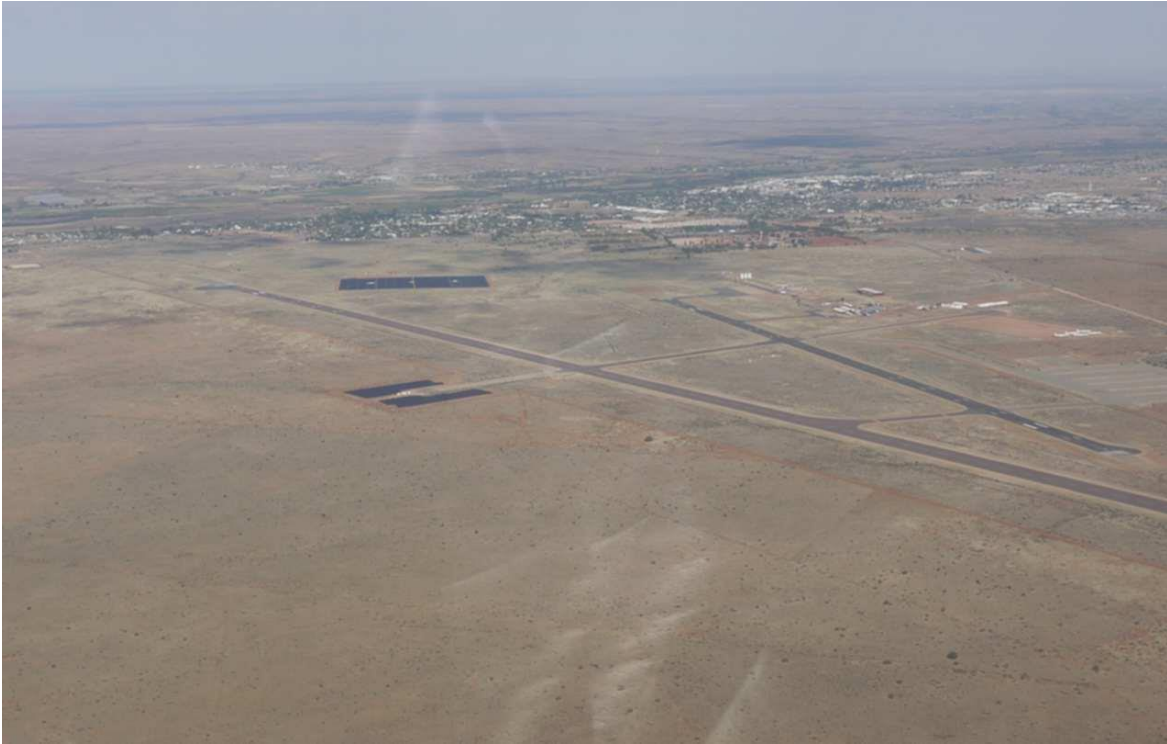
Plate 6, Existing solar arrays at Upington Airport as seen from the air
