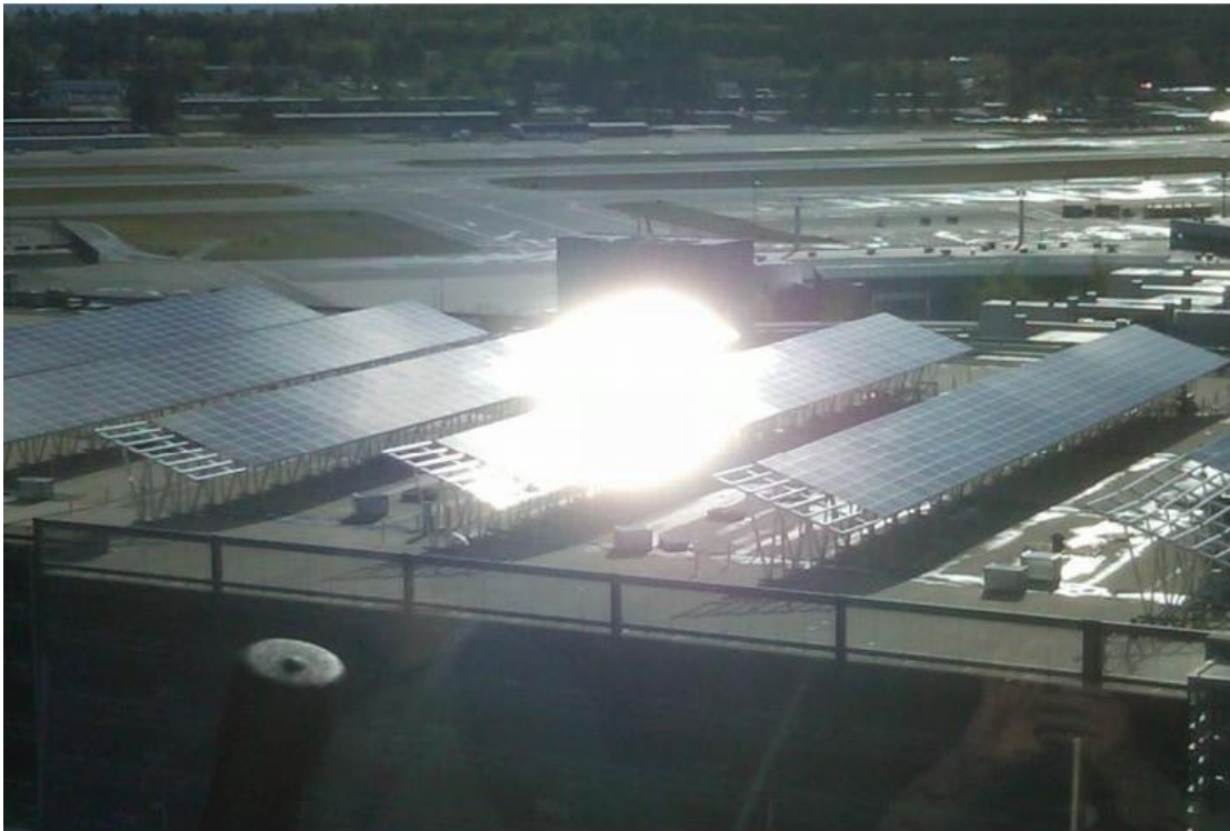
Plate 10 - Glare experienced in the Control Tower at Boston Regional Airport from an adjacent PV array
