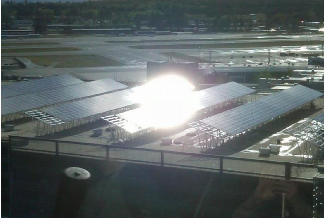
Plate 21 - Glare experienced in the Control Tower at Boston Regional Airport from an adjacent PV array
