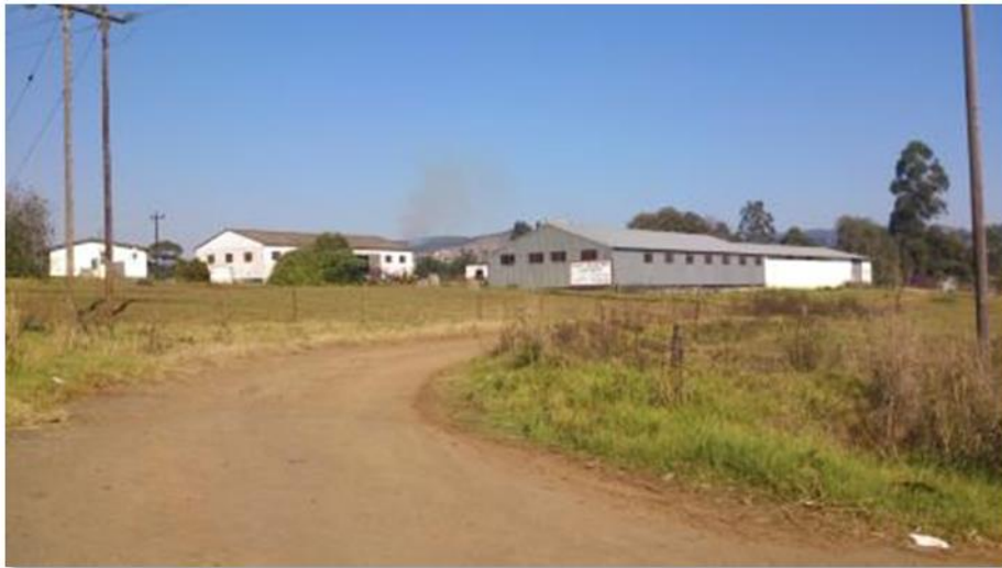
Photograph 2: Existing entrance off the R56 which is to be upgraded. Note the old farm buildings to be demolished.
