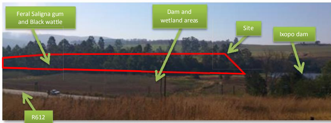
Figure 5: Looking onto site from Ixopo Fresh Produce Market / Tourism Centre
