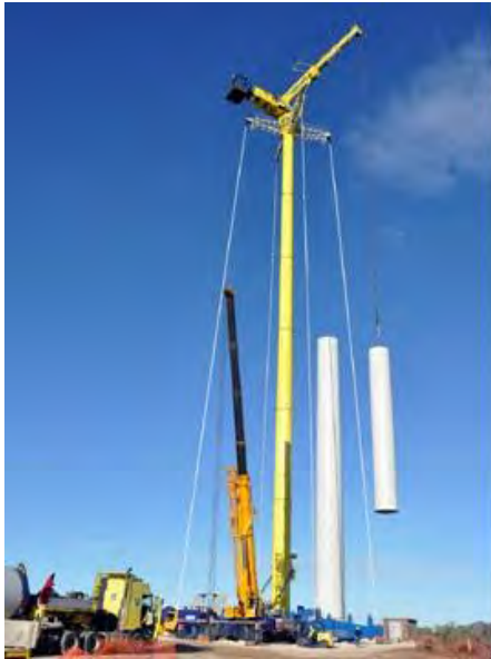
Plate 5: Hydraulic GTK 1100 Crane
