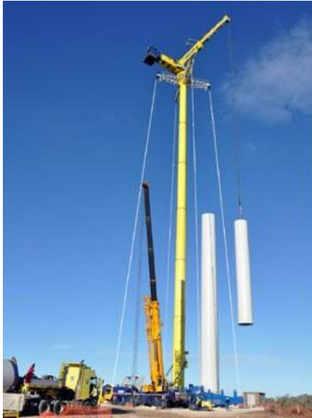
Plate 5: Hydraulic GTK 1100 Crane
