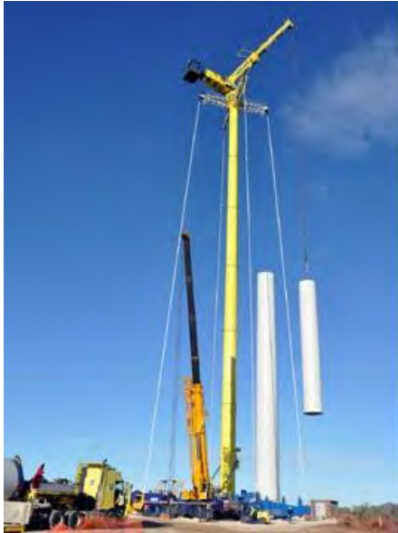
Plate 5: Hydraulic GTK 1100 Crane
