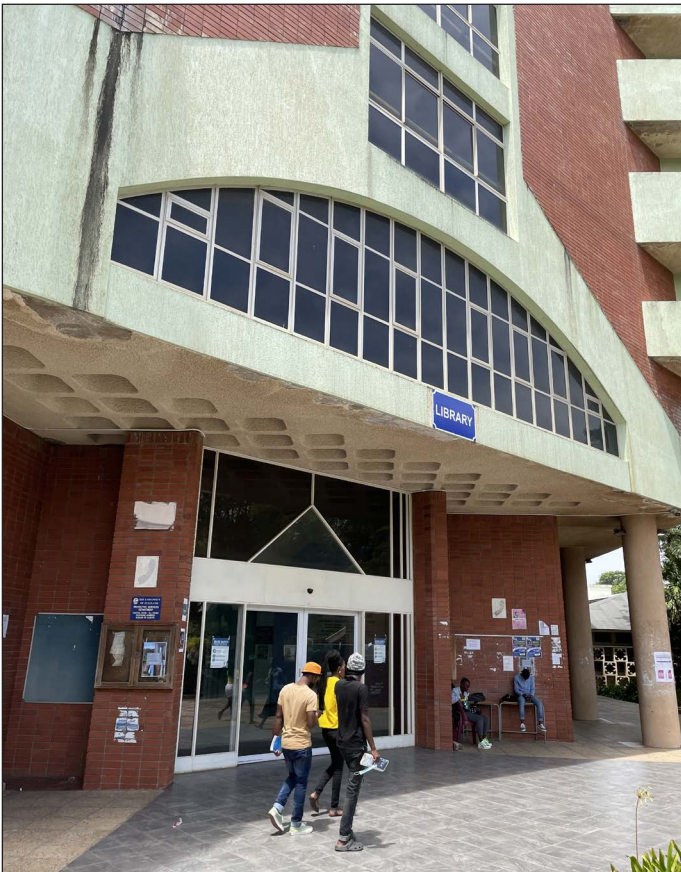
Figure 7T: Library entrance.
