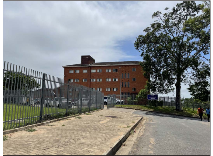
Figure 7V: Residential building, east campus.
