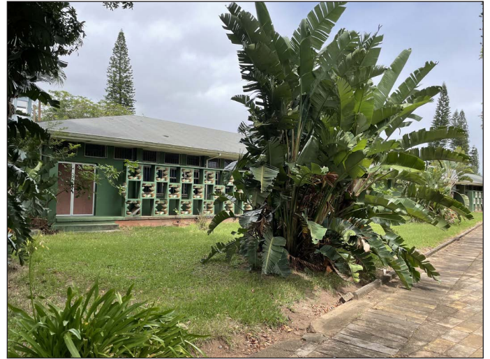
Figure 7H: Original physics block, with original detailing.
