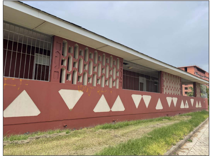
Figure 7b: Warden's house, west residential area, c1960s.
