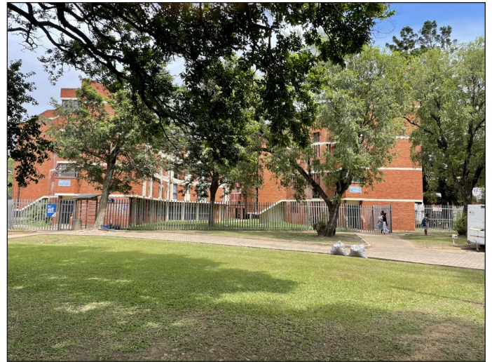
Figure 7d: Residential infill in the west area, c1970s.
