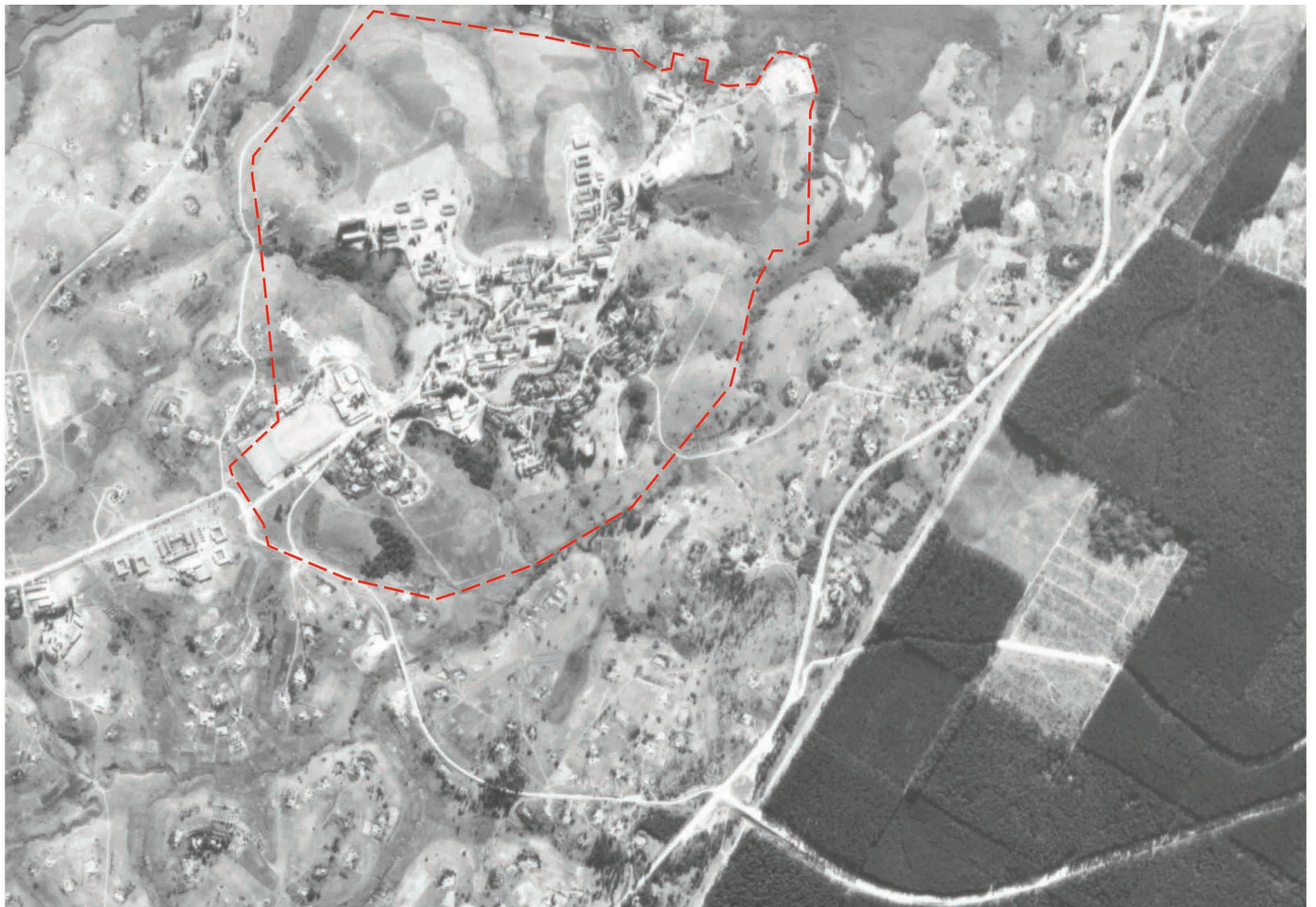
Figure 4D: 1977 aerial photography, showing the infill of more academic buildings on the campus, outlined in red. (Source: NGI Mowbray).
