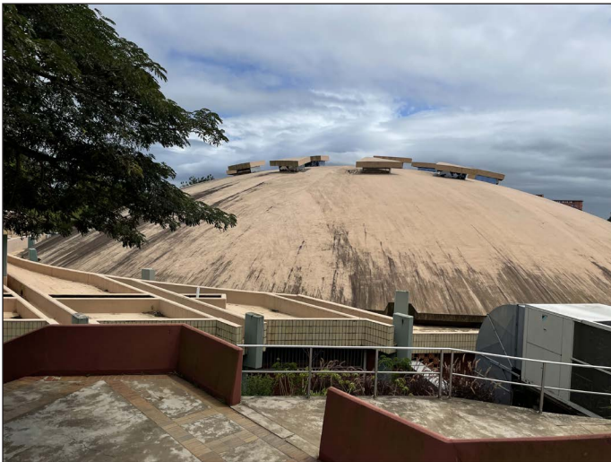
Figure 7M: The King Buthelezi Hall is architecturally interesting.
