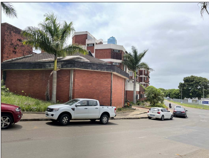
Figure 7O: The southern roadway is more vehicular in orientation.
