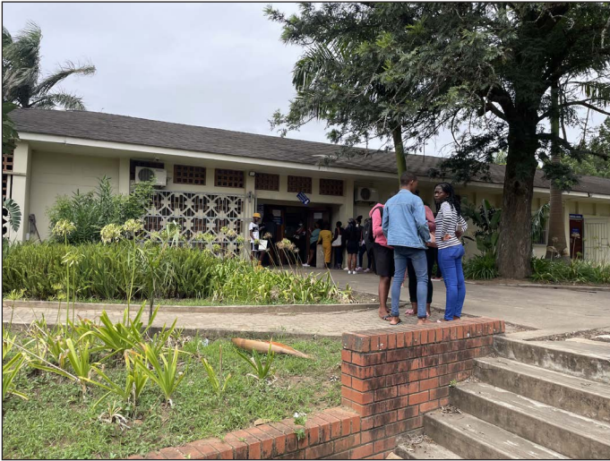
Figure 7G: An original academic buildings, with brise soleil.
