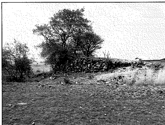
Fig 5: Constructed ramp and support for the lime-burning kiln made by lime workers, which is built in to the thick end of the wedge-shaped loading ramp. The kiln is built so as to enable top loading with alternating layers of fuel and broken limestone, and withdrawal of calcined lime from a drawhole at the base.
