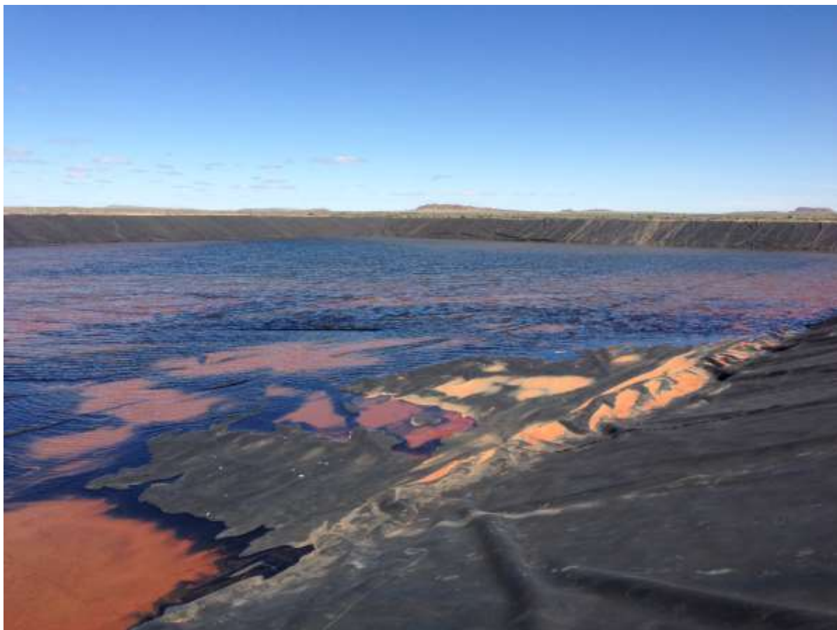
Figure 3.6: Photograph of a typical lined evaporation pond utilised for a CSP Plant
