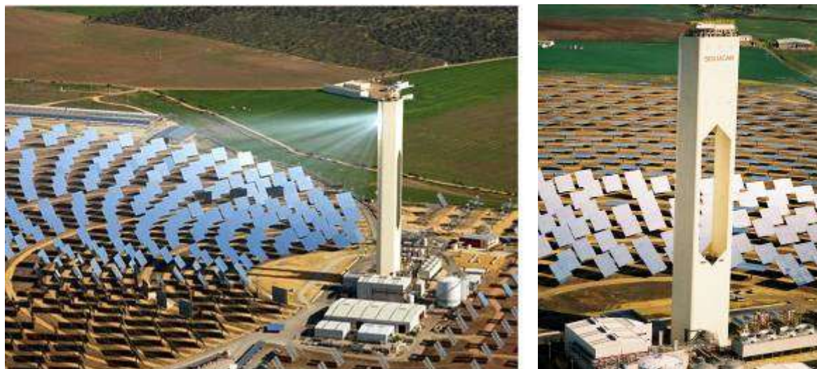
Figure 3.4: Photographs illustrating one of Abengoa Solar’s CSP solar tower plants, courtesy of Abengoa Solar S.A.
