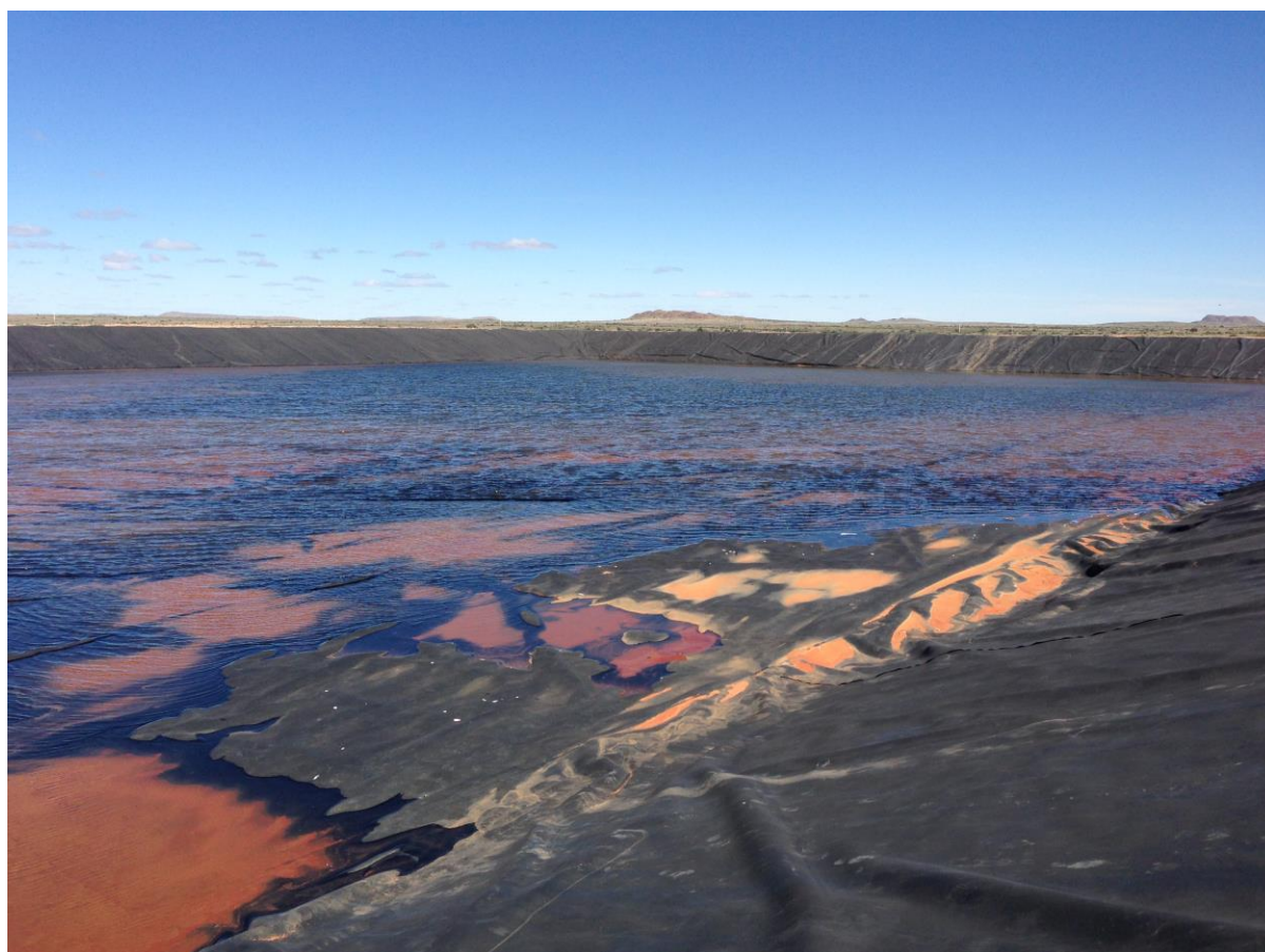
Figure 3.6: Photograph of a typical lined evaporation pond utilised for a CSP Plant
