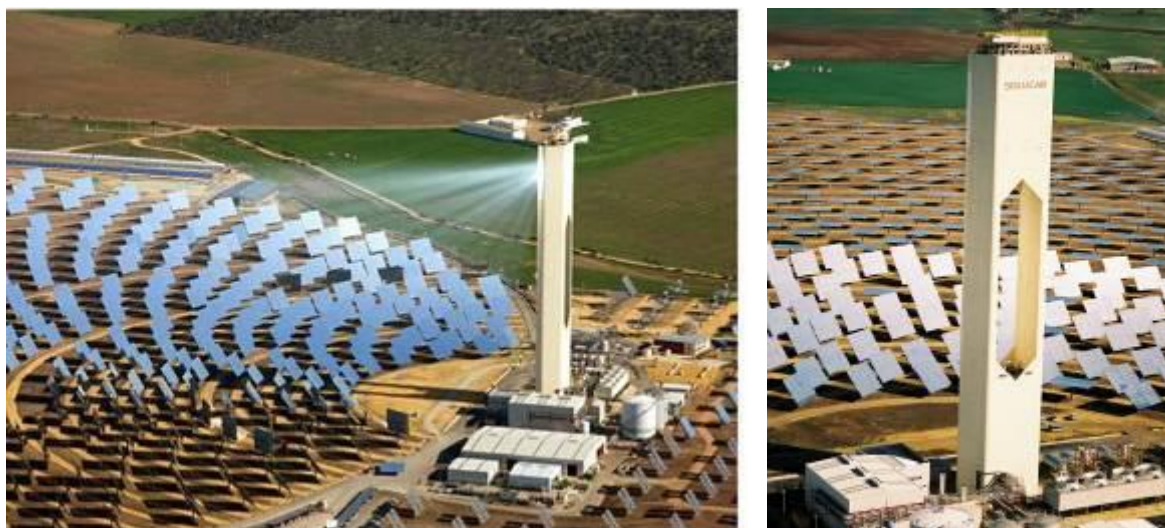
Figure 3.4: Photographs illustrating one of Abengoa Solar's CSP solar tower plants, courtesy of Abengoa Solar S.A.
