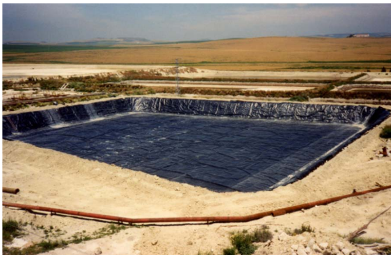
Figure 3.6: Photograph of a typical lined evaporation pond utilised for a CSP Plant
