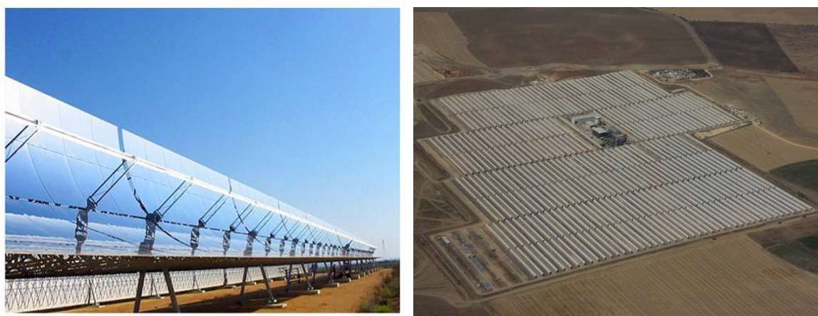
Figure 3.3: Photographs illustrating CSP parabolic troughs plants, courtesy of Abengoa Solar S.A.
