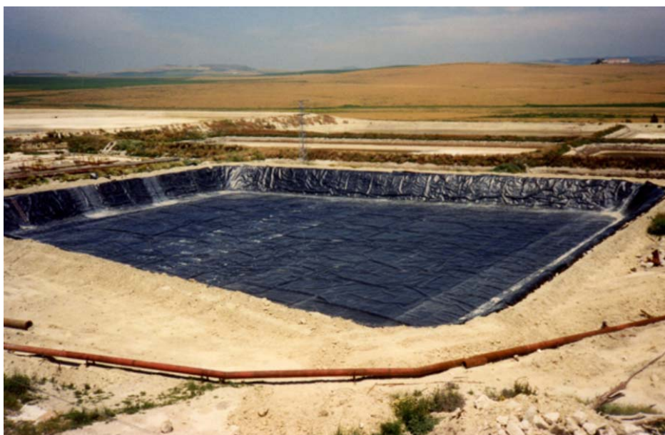
Figure 2.5: Picture of a typical Evaporation Pond utilised for a CSP Plant
