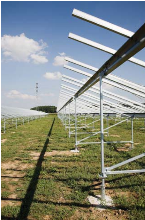
Figure 14. PV plant construction.
