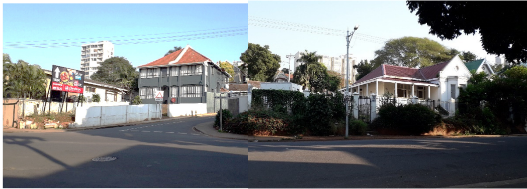
Fig.8, 61 Botanic Avenue and 108 Botanic Gardens Rd Western side of Botanic Gardens Rd (opposite no. 99-105). Residences set-back from the road and above the road, accessed off Botanic Avenue.
