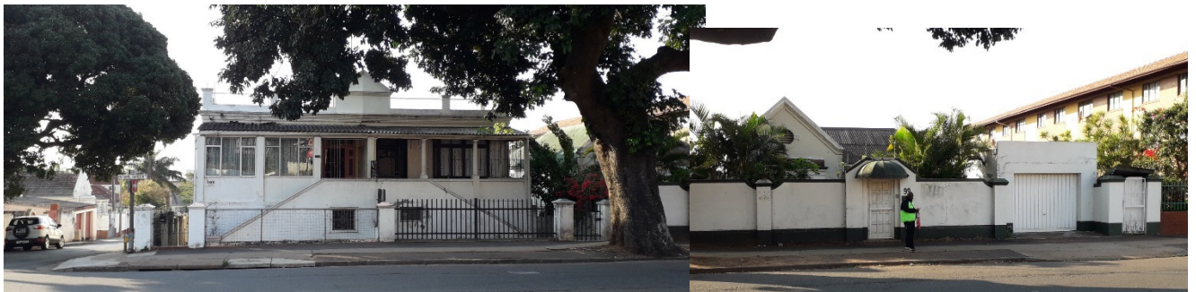
Fig.9, 99-105 Botanic Gardens Rd (Eastern side of Botanic Gardens Rd) No. 105 and 101 are a pair of semi-detached houses, situated on the corner of Botanic Avenue with entrance level raised a half-storey above the street, resulting in a 1.5 storey building on the street. The boundary is defined with piers and a fence on Botanic Gardens Rd and a solid wall on Botanic Avenue. No.99 is a single-storey house situated lower than the street, garage and boundary wall screen the veranda and gable from view. A three-storey (1970's) residential block is adjacent to the South.
