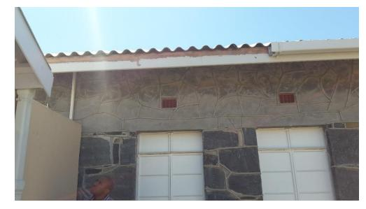
3. Replace broken asbestos gutter with fiber cement approx. 3 linear Meters
