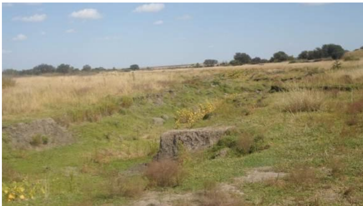
Image 5: Dongas on the North Western side of the dam on farm Doorndraai East 235
