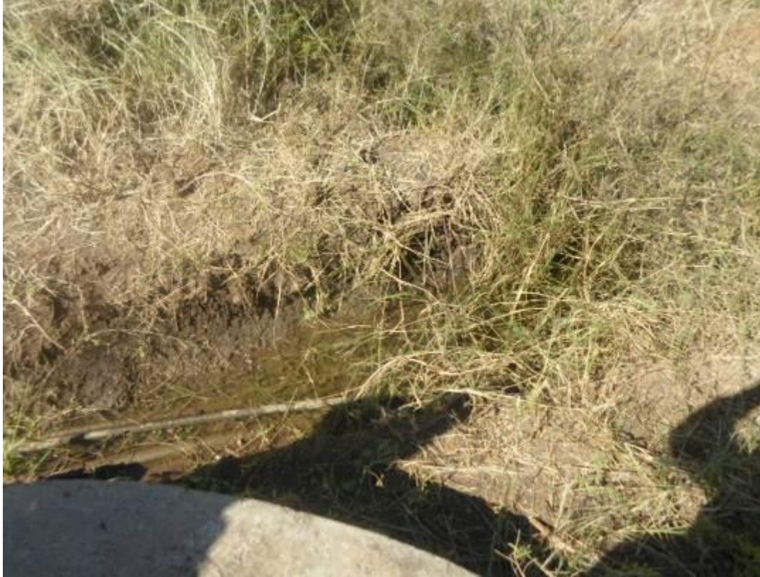
Image 19: Pipeline on farm Thornvale 147 in close proximity of proposed transformer pole number VM88-86-152-44
