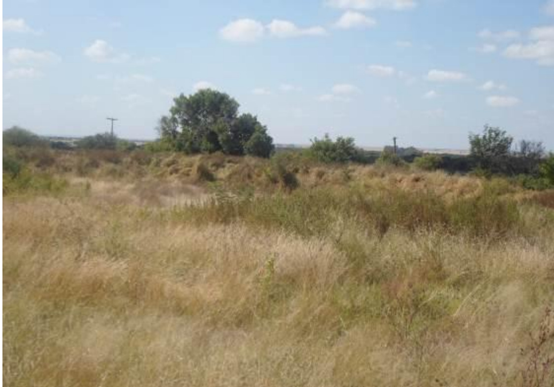
Image 3: Man-made dam wall on farm Doorndraai East 235
