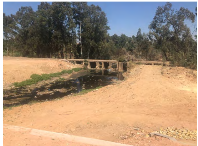
Figure 7-59 - View of old Crownwood road bridge
