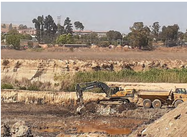
Example of excavators working to remove silt.
