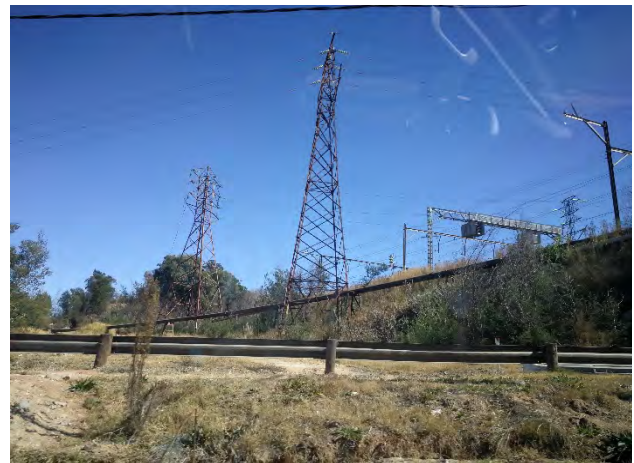
Figure 1-4: Infrastructure found in the project area including pipelines and powerlines.
