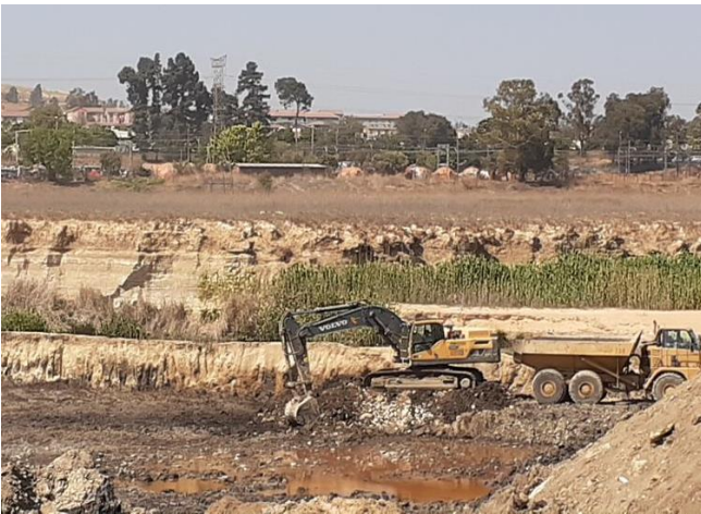
Example of excavators working to remove silt.
