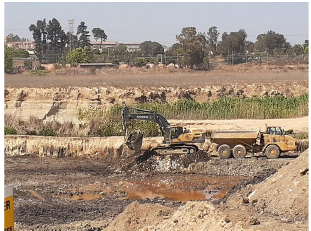
Example of silt being loaded from the watercourse onto a ADT
