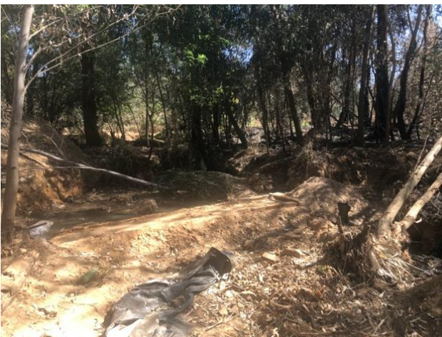
Figure 7-44 - Illegal mining activity close to Crown Mines
