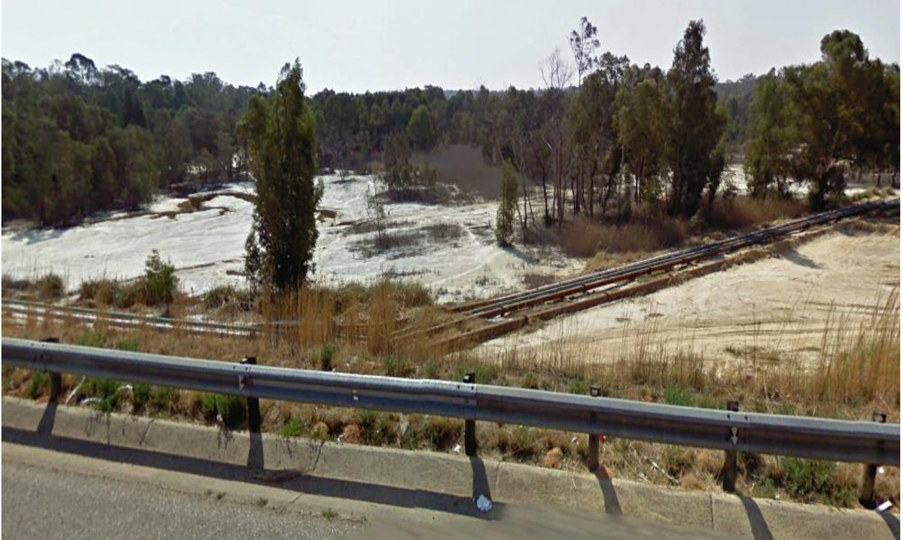
Figure 1-7: A portion of the Russell Stream which will be excavated. This image was taken at the following location: 26°13'46.58"S; 27°59'43.03"E
