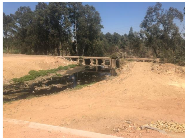
Figure 7-45 - View of old Crownwood road bridge
