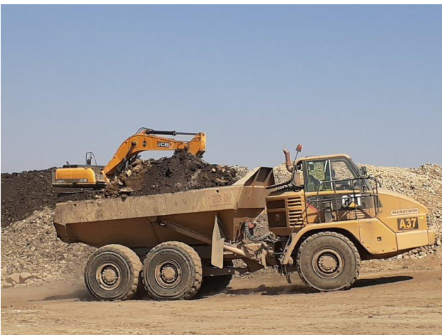
Example of new silts being transported for stockpiling
