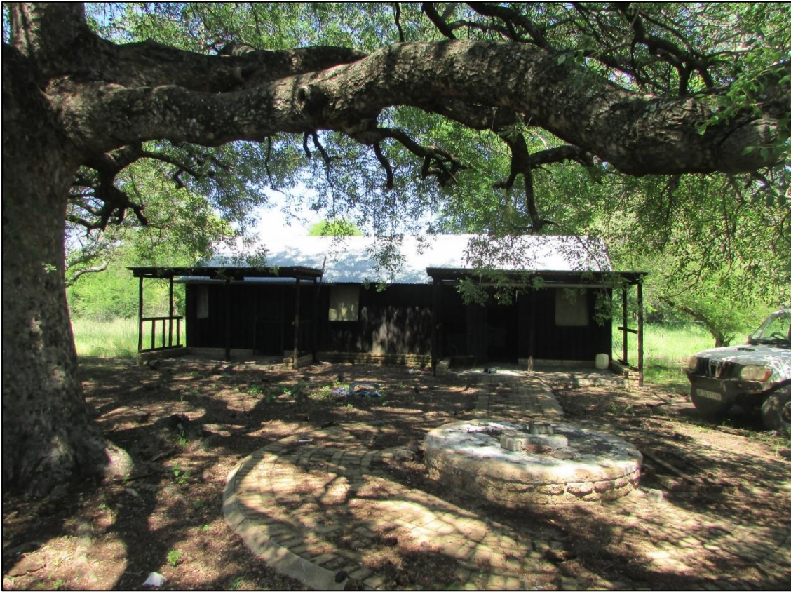
Figure 5.32: View of the Bush Camp on the Farm Tusschenkomst (Site 5)
