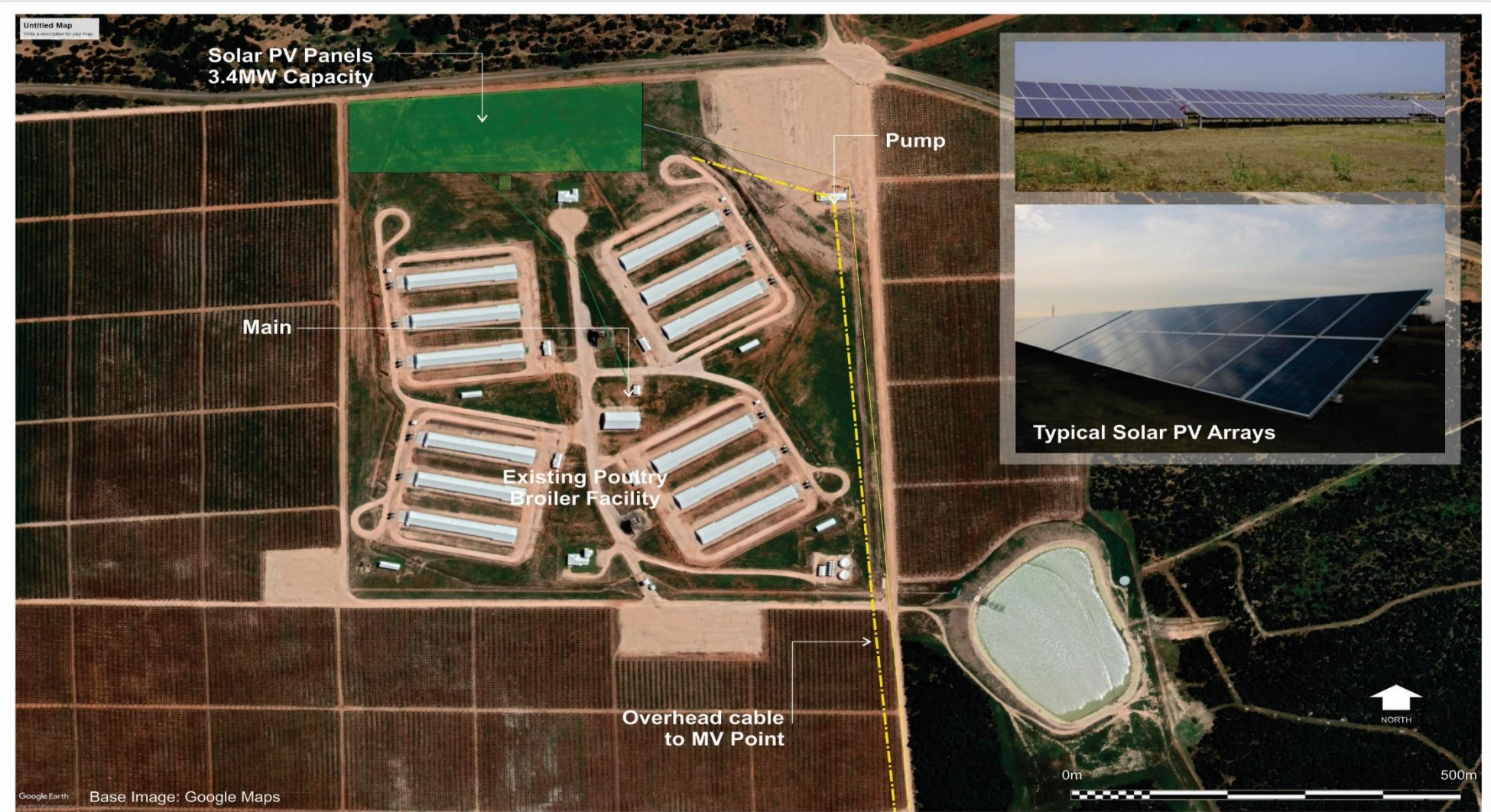
Figure 03: CONTEXT- Disco 2 PV Solar Facility
