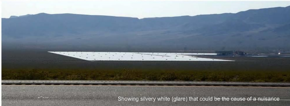
Apparent colour changes with differing sun angles and viewing geometry at a PV facility. (USDI 2013:78) Credit: Robert Sullivan, Agganne National Laboratory.
