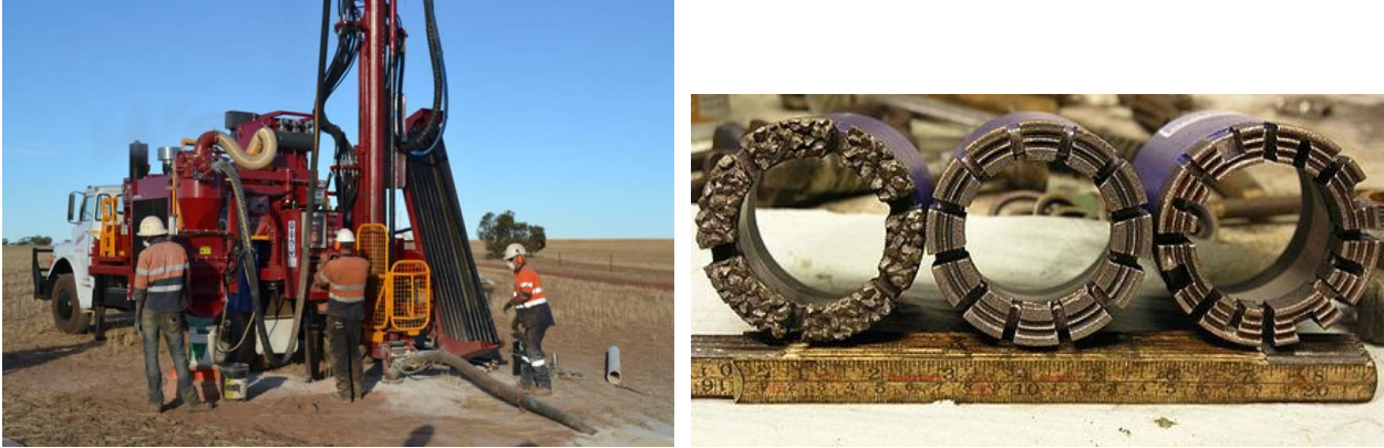
Figure 7: Drilling setting and equipment
