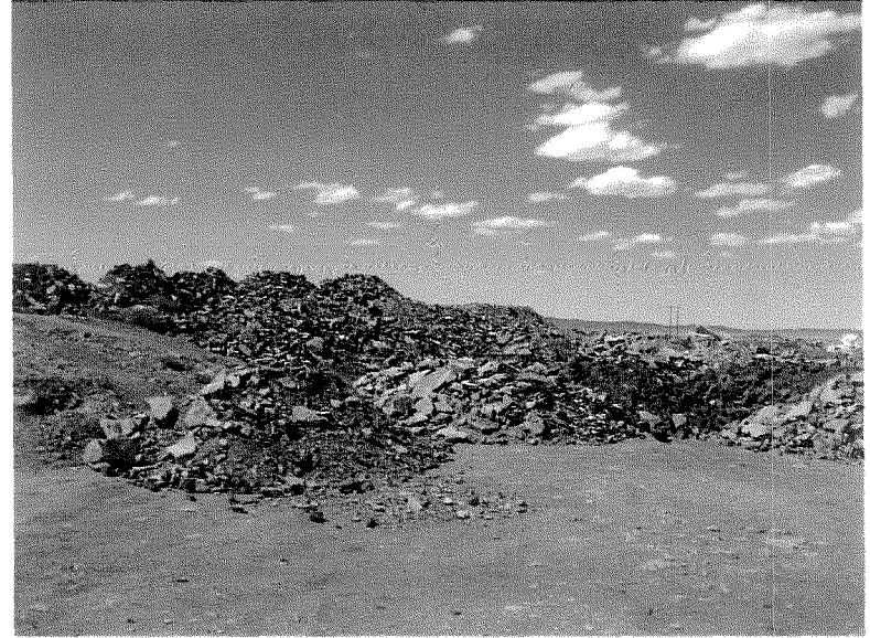
Plate C1.2 Excavated material stockpiles adjacent to the proposed borrow pit area. Photograph taken looking northeast.
