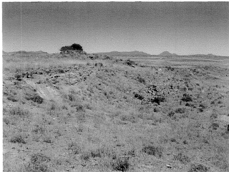
Plate C8.3 Photograph taken from the southeastern edge of the borrow pit looking south.
