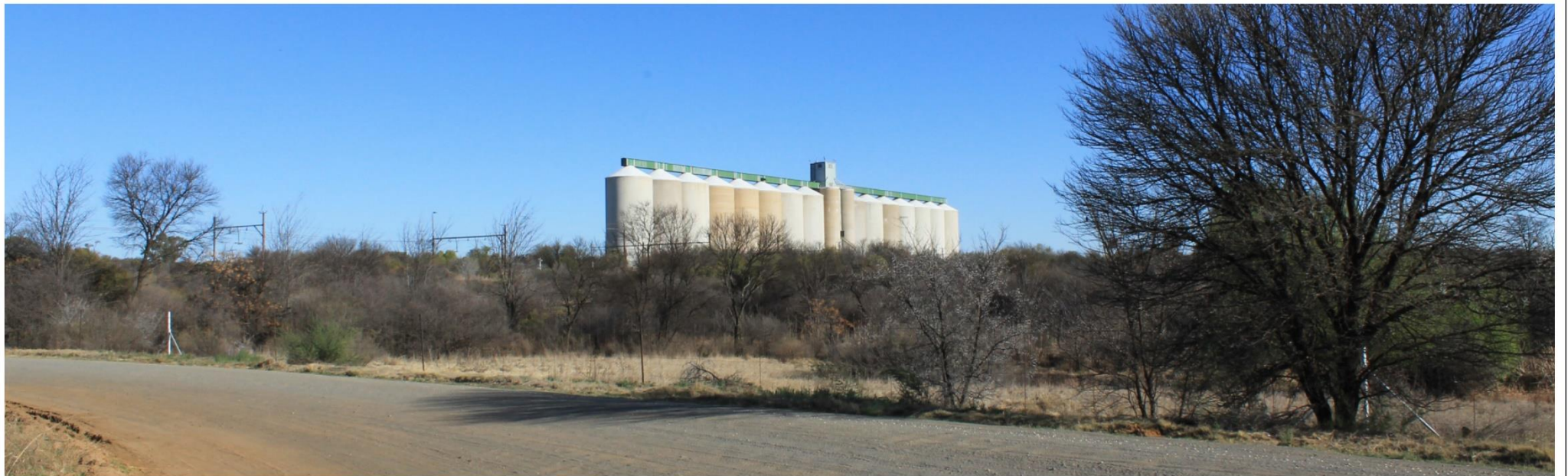
CL 34 along S484, looking South. Note: Senwest Grainlink agricultural silos.
