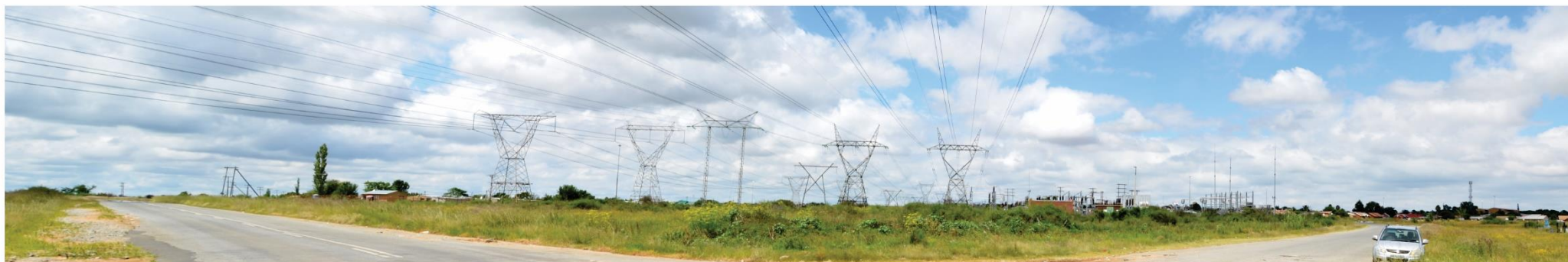
CL 237 looking northwest towards the existing substation at the entrance to the township of Meloding
