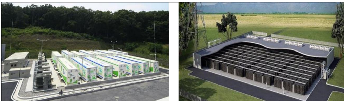
Figure 8. Battery Energy Storage System (BESS)
