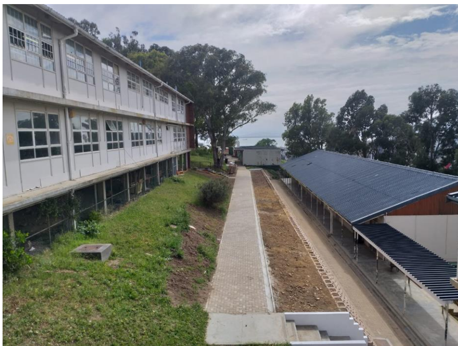
Figure 12B after: new paving at upper tier.
