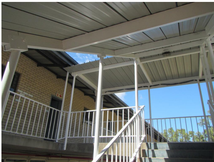
Figure 15B after: Balustrades and handrails sanded, treated, and painted white.
