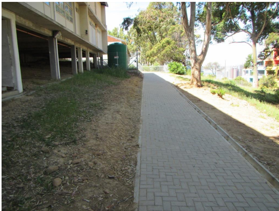
Figure 14C after: new paving/walkway at lower tier
