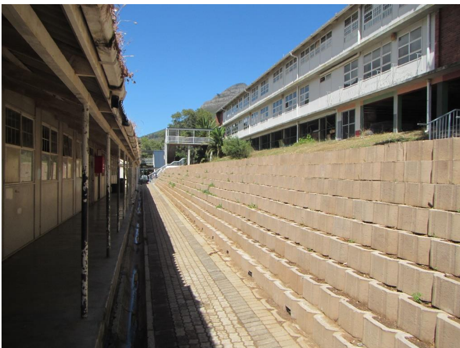
Figure 13B after: new retaining wall at upper tier.
