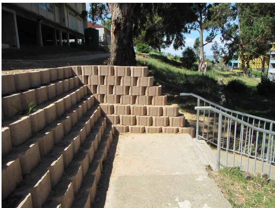
Figure 14B after: new retaining wall at lower tier (entrance walkway).
