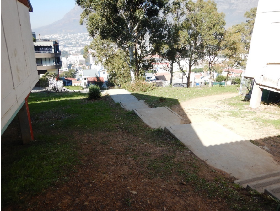
Figure 4.6: Staircase 2 (see site plan) – to receive safety handrails on both sides.
