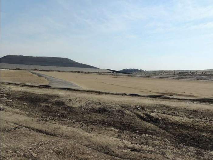
Figure 7: Pollution Control Dam at Class-A waste facility
