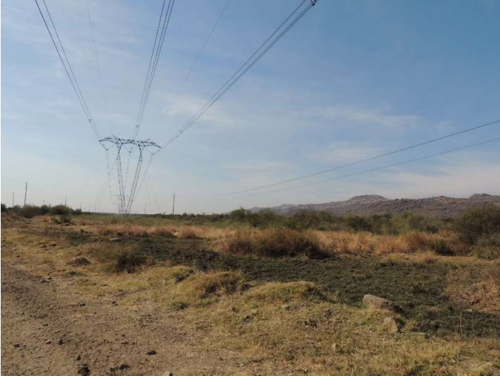
The view from the southern side of the mine
