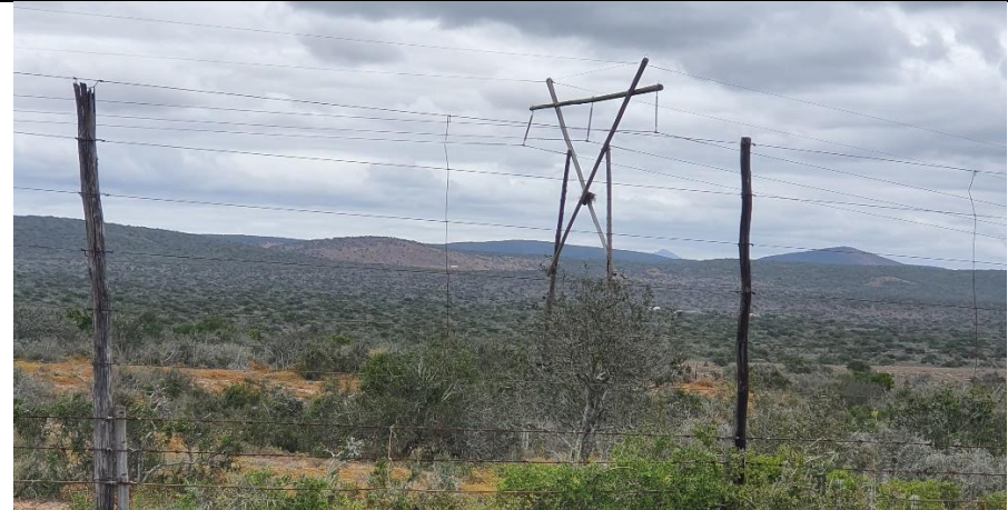
Pylons and powerlines routed adjacent to the R75 road
