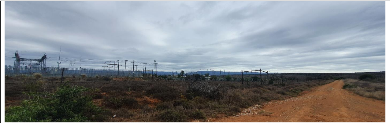
Viewpoint 4: Farm Road and Skilpad Substation– looking west. The project will be highly visible in the foreground.
