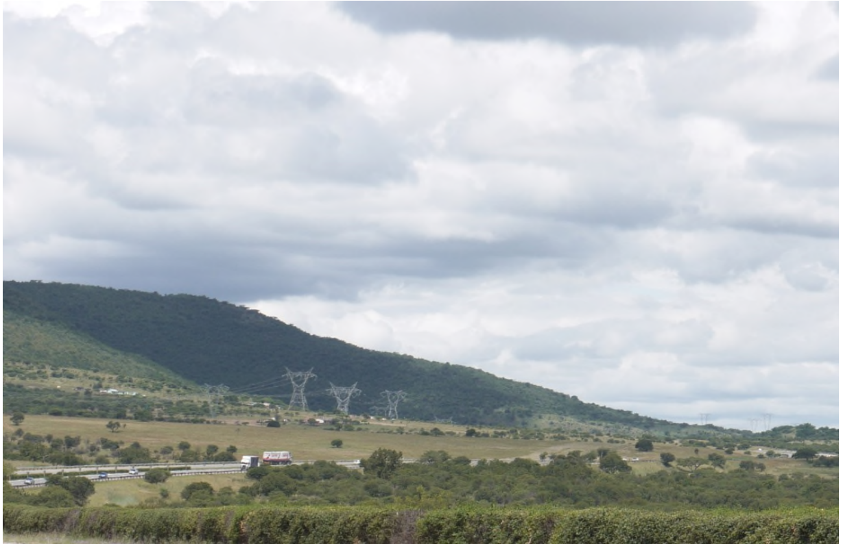
Plate 13 - 400kV double overhead transmission lines. Pylons are obvious in the mid distance (approximately 2-3km) but are not highly conspicuous at a distance (approximately 5-6km) as they cross the ridgeline.
