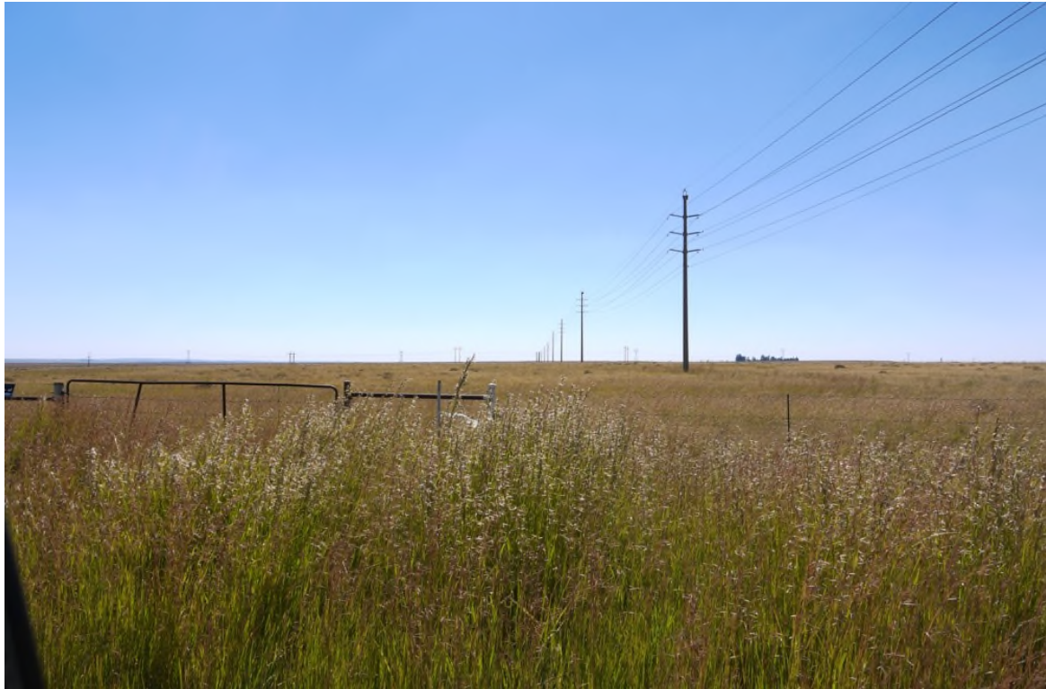
Plate 12. A view along the line of a 132kV overhead power line with monopole towers.
