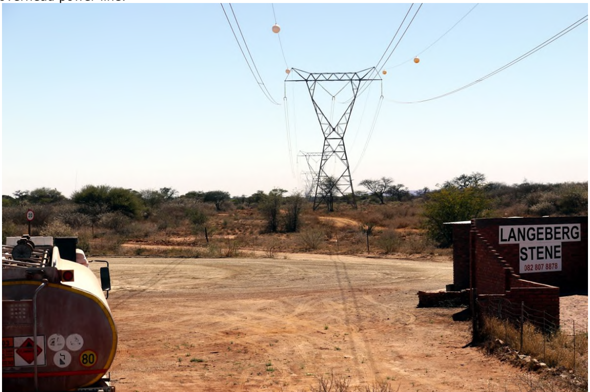
Plate 20 - VP5 located on the N14 at the crossing point of the existing 400kV overhead power line looking north east along the line.
