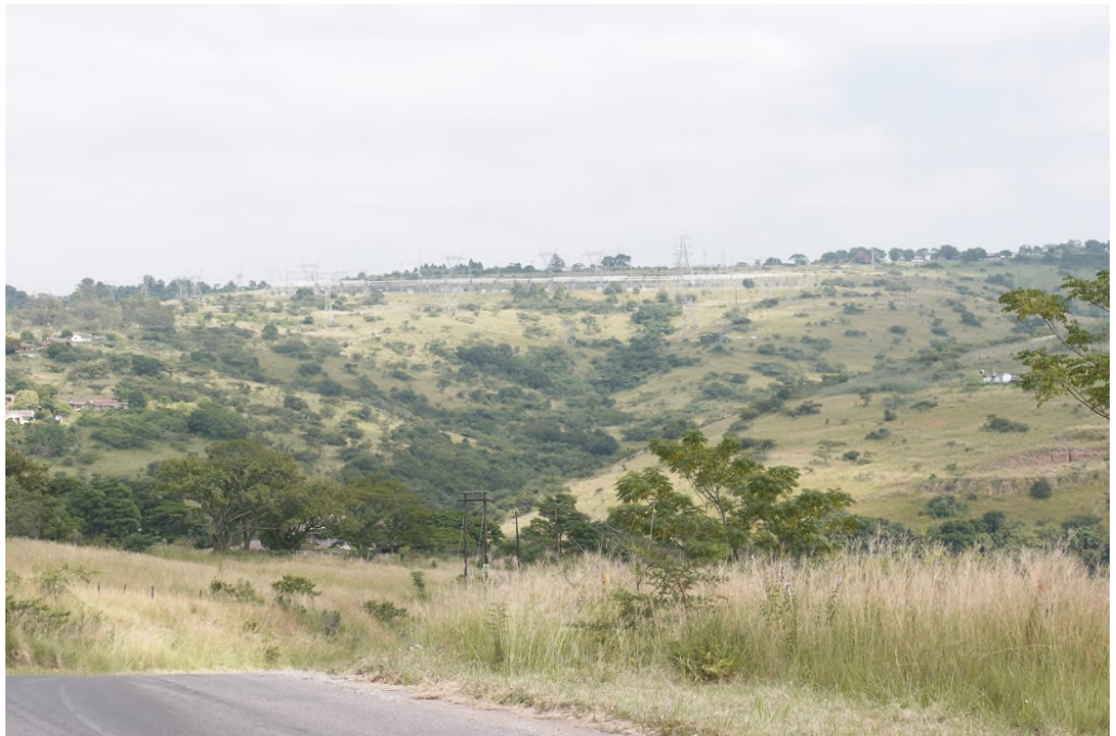
Plate 15, Distance view (1.5-2.0km) of the existing Hammersdale 400kV Sub Station. Note the 400kV pylons entering the site are the most obvious elements
