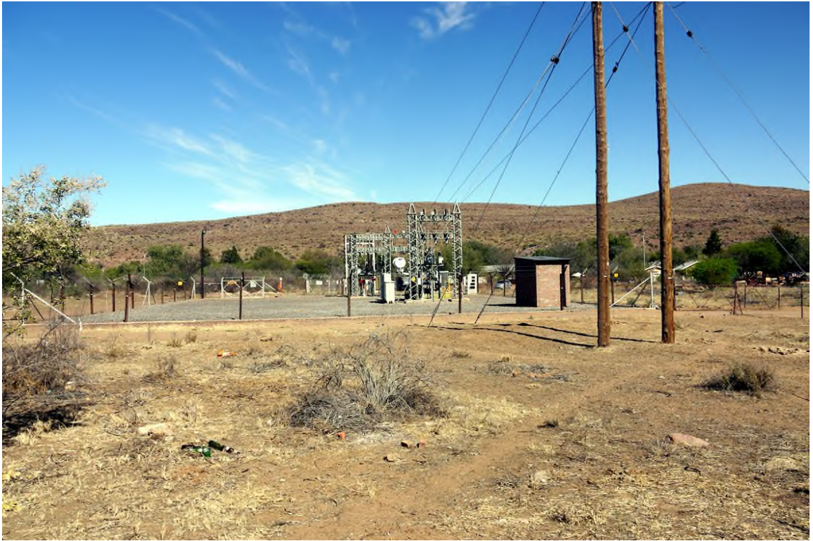
Plate 25 – VP10 looking west towards the existing substation.
