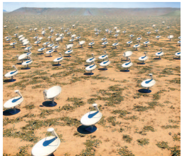
Figures 3a and 3b: Illustration of Meerkat dish antenna. Height 19.5m and dish 13.5m diameter.
