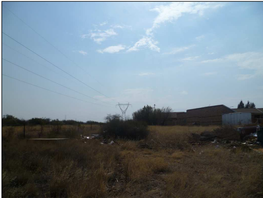
Figure 14: View of the existing 132kV power line within corridor alternative 1A. Note the residential dwellings at Lime Acres within the corridor.
