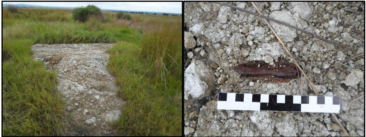
Figure 41. General site conditions at VF1.
