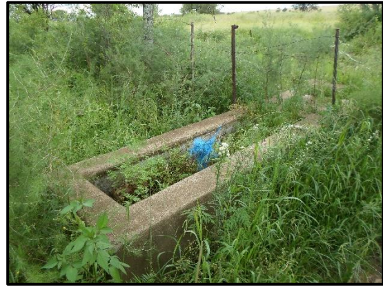
Figure 35. Site conditions at S3.
