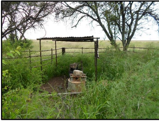
Figure 34. Site conditions at S3.
