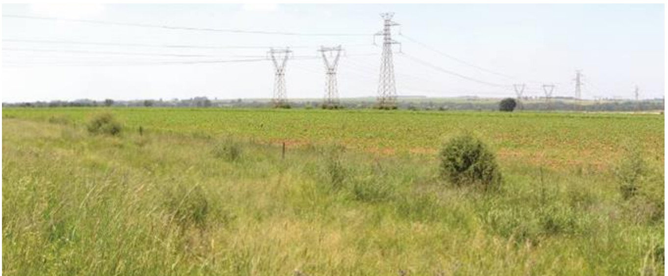
FIGURE 8: VIEW OF EXISTING POWERLINES LOCATED WITHIN THE STUDY AREA.
