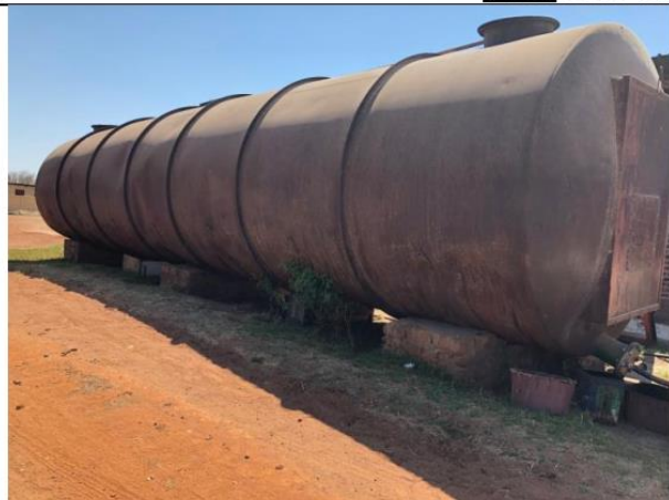
Molasses storage tank
