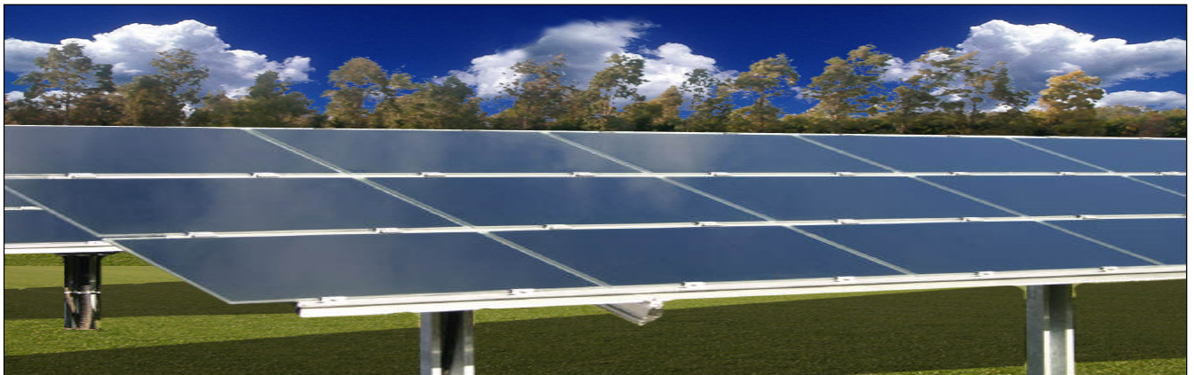
Figure 5: Frontal view of PV arrays mounted on fixed mounting systems
