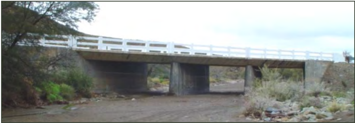
Figure 7: Elevation view of typical bridge on R354
