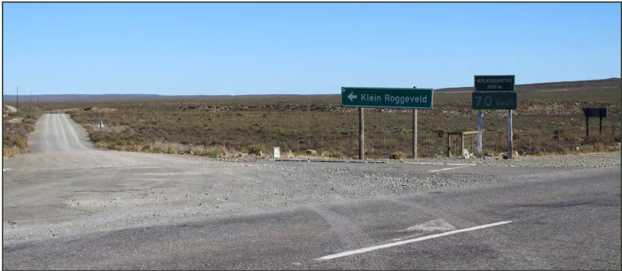
Figure 10: Klein Roggeveld turn-off
