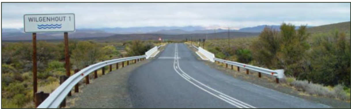
Figure 8: Approach view of typical bridge on R354
