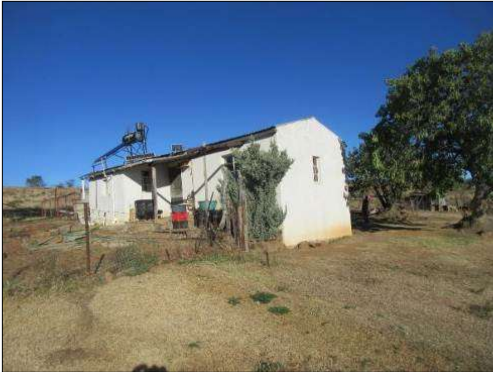
Photograph 7.6: Labourer's house on Highlands Farm
