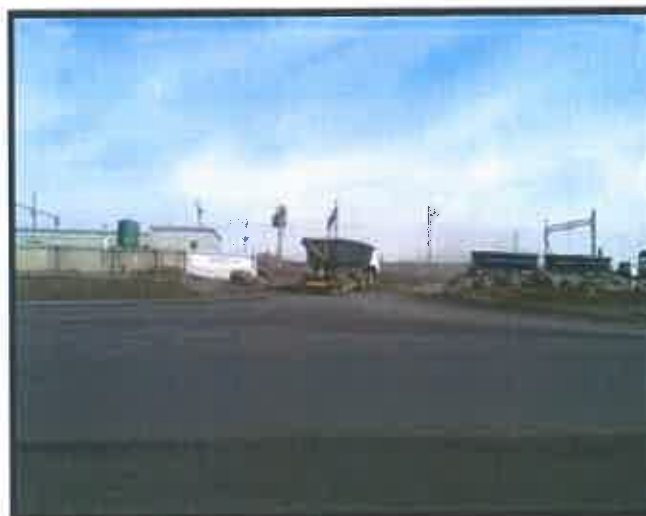
Photograph 2.2-2: View of Site Activities
