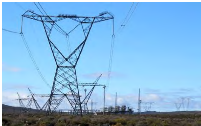
Plate 8-10: Existing power lines and substation to the south of the site.
