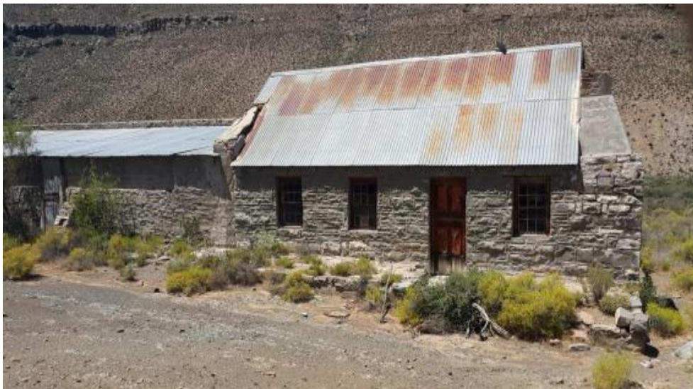
Plate 8-7: Farm buildings at Venters Rivier. Small 19th century dwelling house, joinery is intact. Note the large vernacular style hearth and barn (waenhuis) appended onto the gable end.
