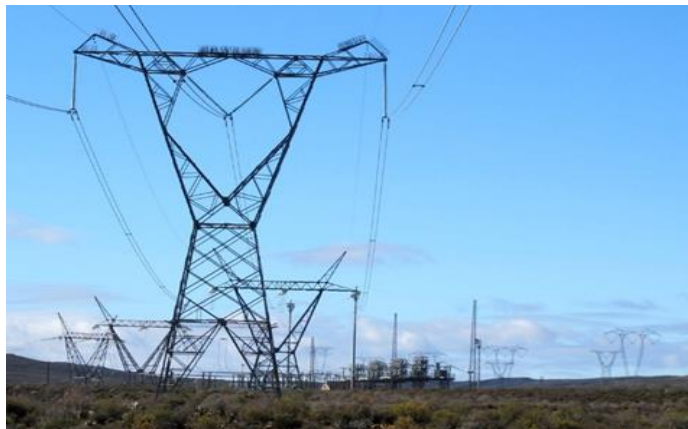
Plate 8-13: Existing power lines and substation to the south of the site.
