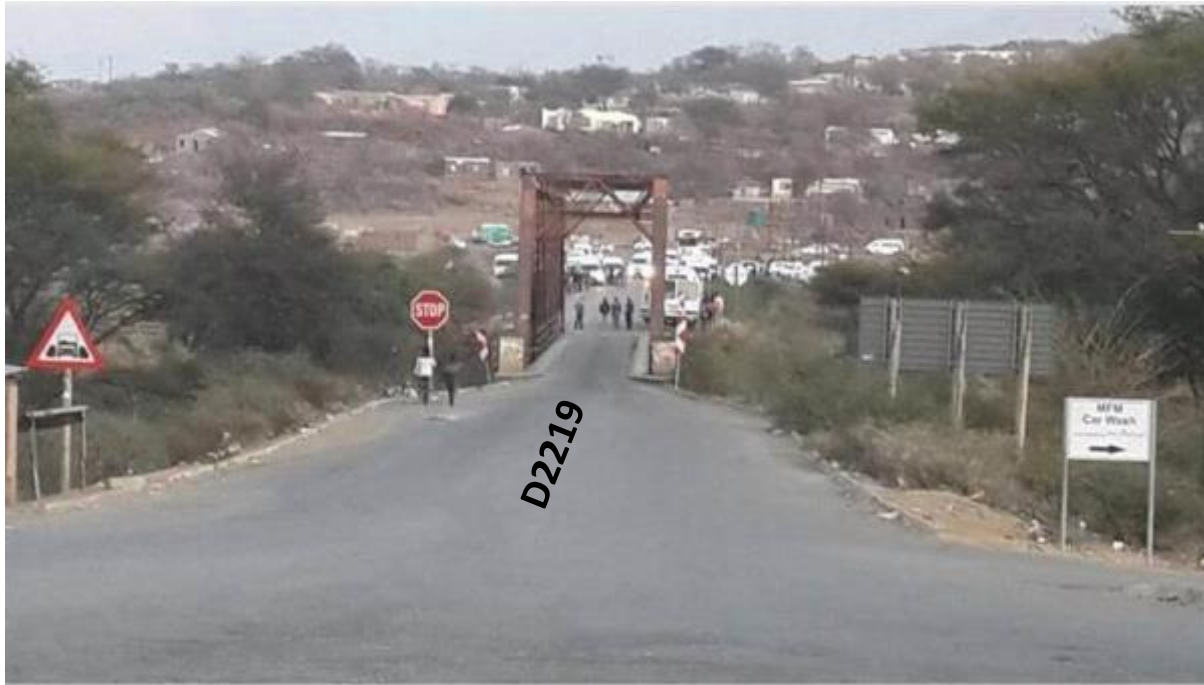
Figure 74: Malekane Steel Bridge
