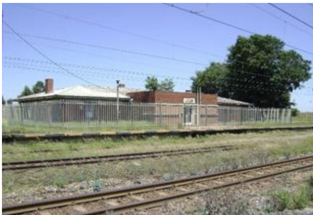
Figure 16.2-1: Front view of the Old station building
