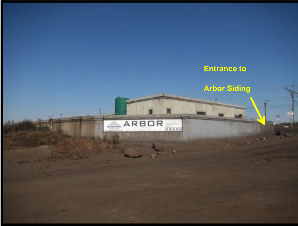
Photograph 7.1-18: The entrance to the Arbor Siding on the R555 road towards Delmas.
