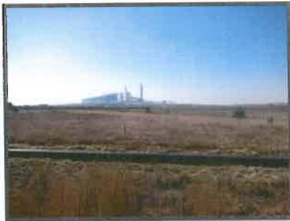
Photograph 3.1-6: Eskom Kusile Power Station north east of the Arbor Siding
