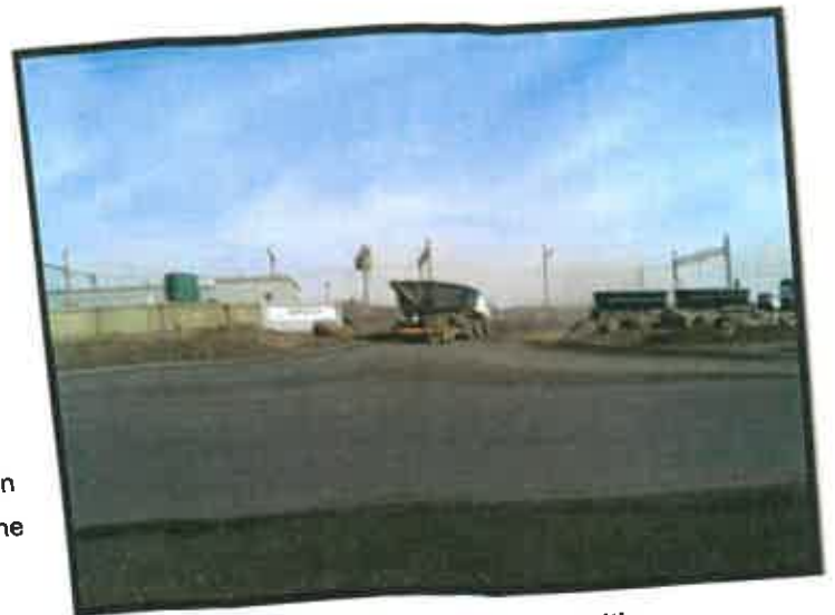
Photograph 2.2-2: View of Site Activities
