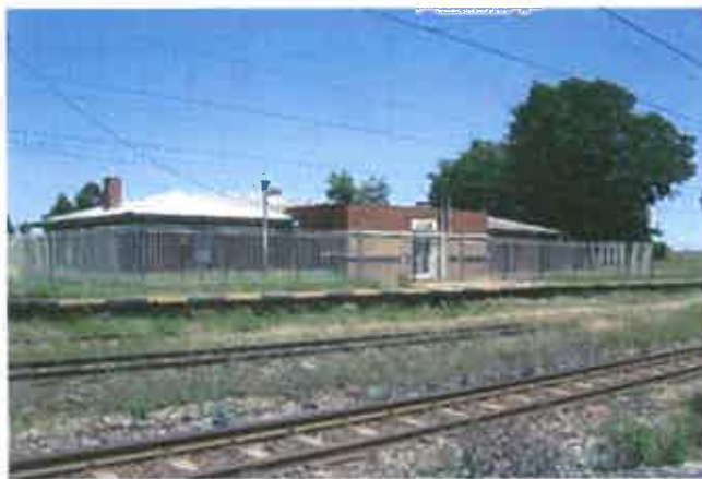
Figure 16.2-1: Front view of the Old station building
