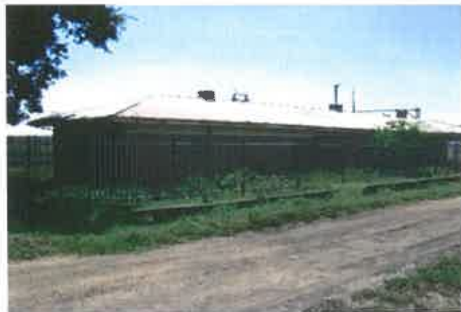
Figure 16.2-2: Rear view of the Old station building Impact assessment
