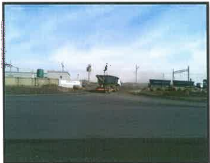
Photograph 2.2-2: View of Site Activities
