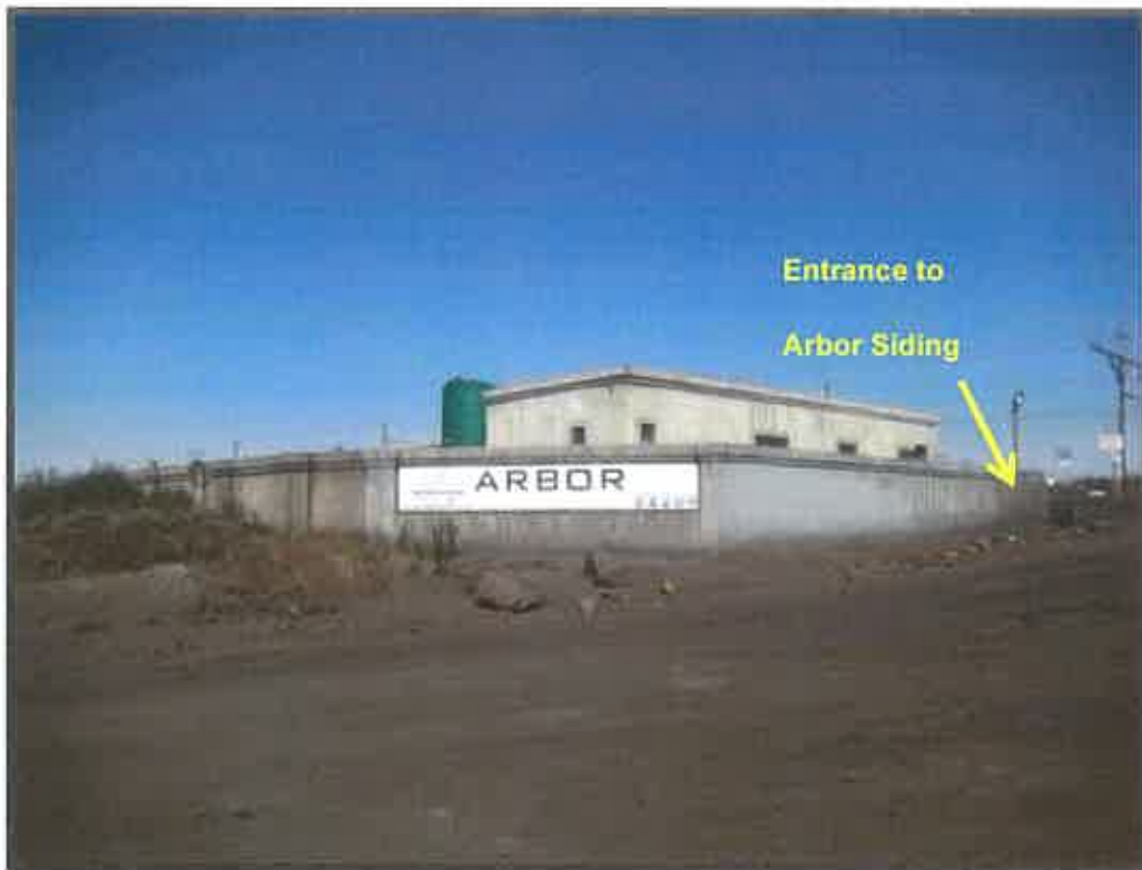
Photograph 7.1-18: The entrance to the Arbor Siding on the R555 road towards Delmas.
