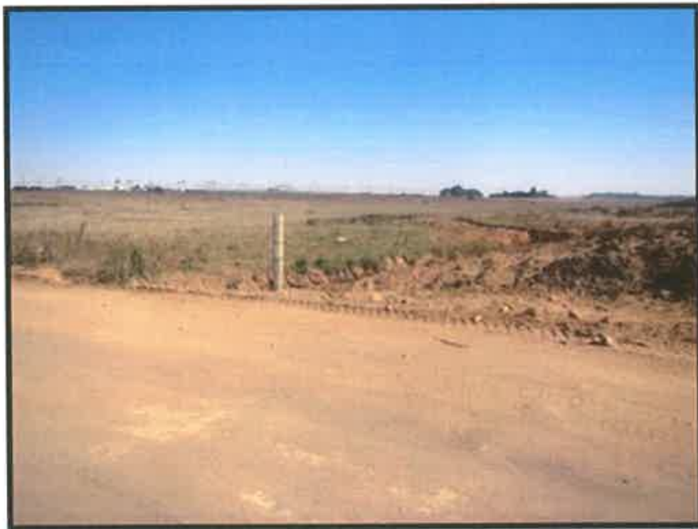
Photograph 7.1-15: The road works by the Mpumalanga Provincial Government Department of Public Works, Roads and Transport in Nkangala have created a visual intrusion and impeding on the wetland with the disposal of soil and rubble on the edges of the as wetland (north east side) (26° 02' 097" S; 0,28° 53' 027" E).
