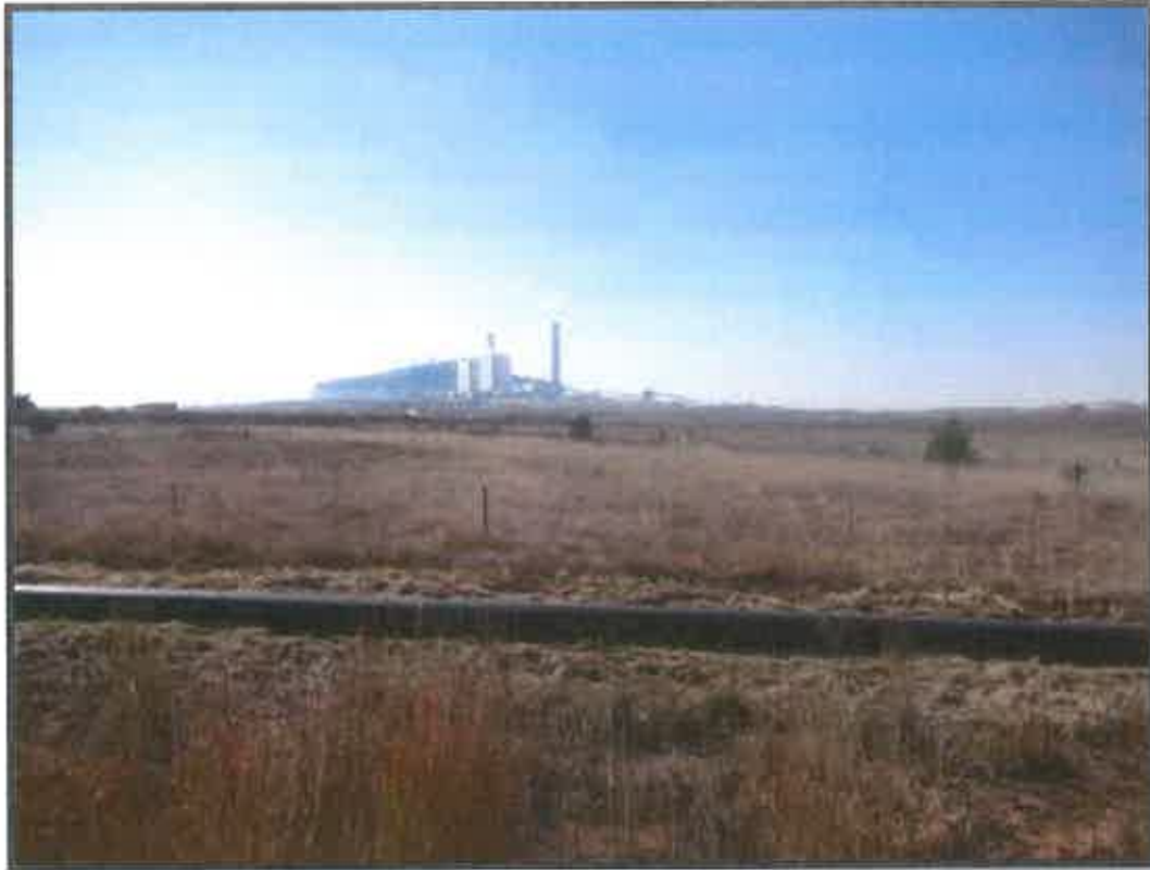
Photograph 7.1-8: Kusile Power Station north east of the Arbor Siding (25° 59' 073" S; 0,28° 53' 063" E).
