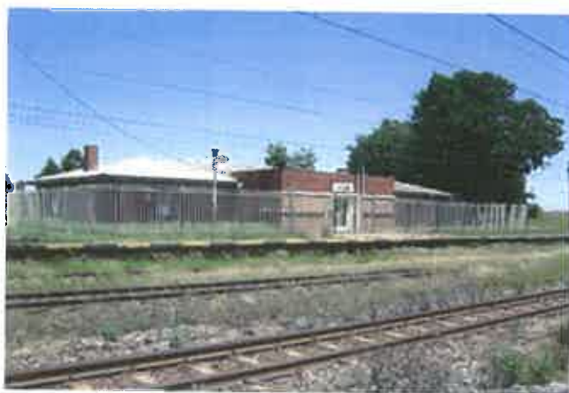
Figure 16.2-1: Front view of the Old station building
