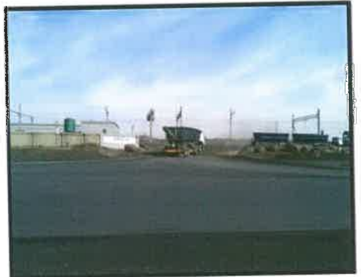
Photograph 2.2-2: View of Site Activities
