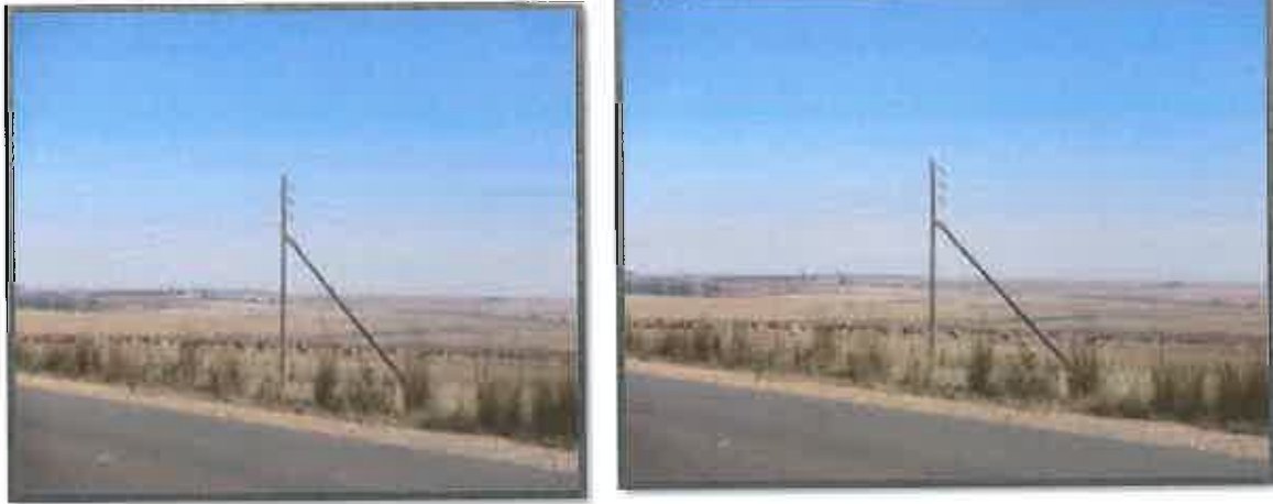
Photograph 7.1-12: Road infrastructure upgrade by the Mpumalanga Provincial Government Department of Public Works, Roads and Transport in Nkangala (26° 01' 118" S; 0,28° 53' 058" E).
