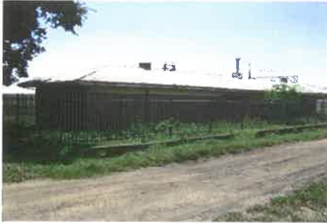
Figure 16.2-2: Rear view of the Old station building
