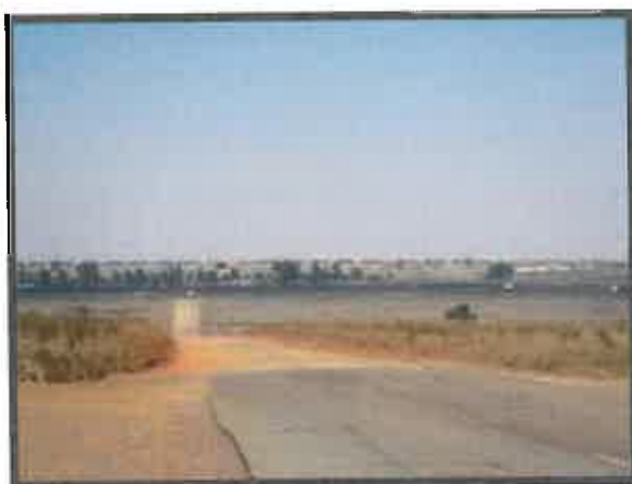
Photograph 3.1-7: The view of the Arbor Railway Siding. The beginning of the gravel road stretch towards the site
