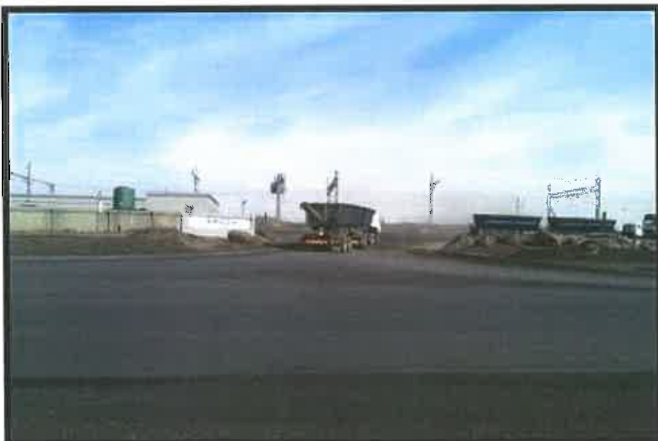
Photograph 6.1-2: View of Site Activities
