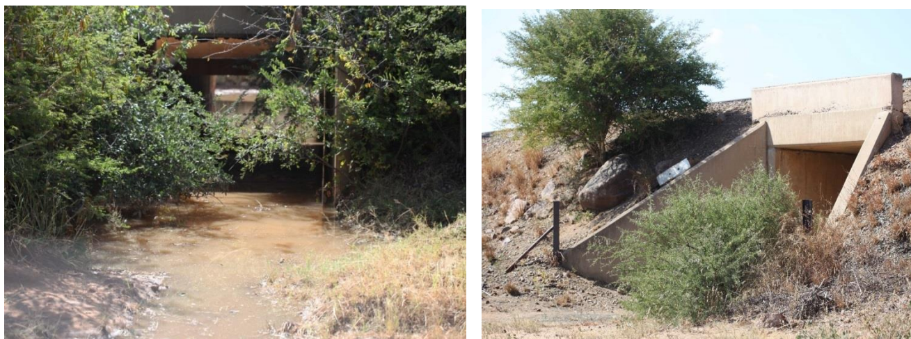
Figure 20: (Left) Culvert of Streamcrossing No. 3 at the site. Water visible in picture gathered after substantial rains (RF. Terblanche, 2019) during Summer Survey. (Right) Culvert of Streamcrossing No. 1 at the site during winter. The non-perennial stream is dried up confirming the attenuation of water at the site is dependent on rainfall events.
