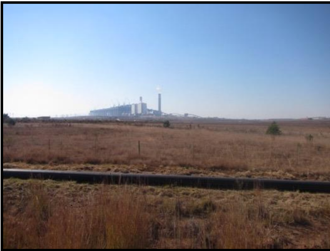
Photograph 9.1-8: Kusile Power Station north east of the Arbor Siding (25° 59' 073" S; 0,28° 53' 063" E).
