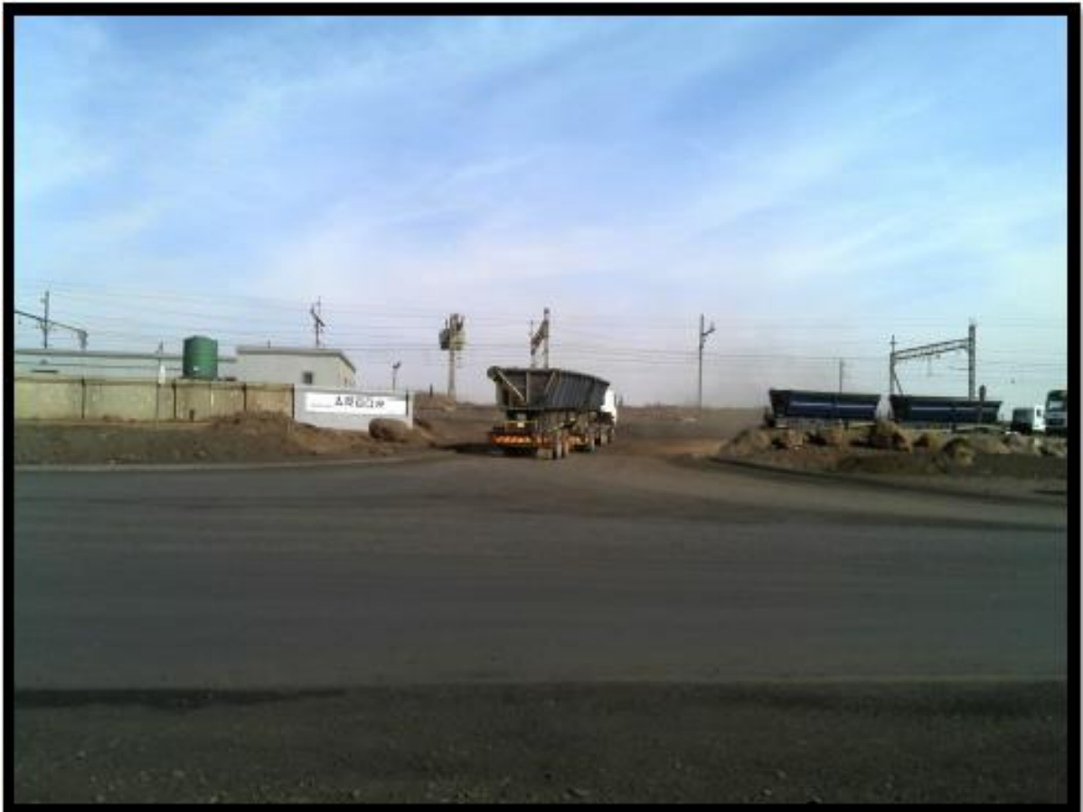
Photograph 3.1-1: View of Site Activities
