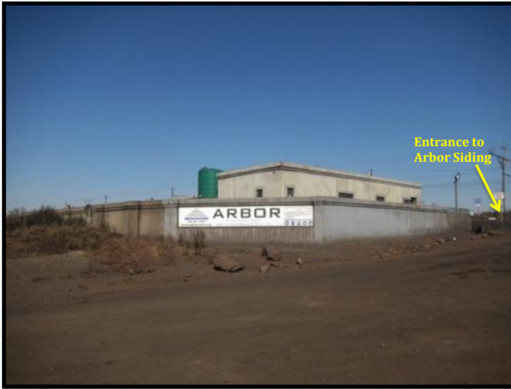
Photograph 9.1-18: The entrance to the Arbor Siding on the R555 road towards Delmas.
